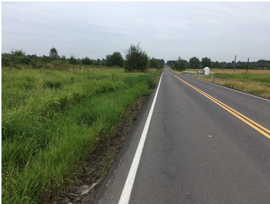
Figure 1: NW 38 th Avenue at Grass Valley Park, facing west
