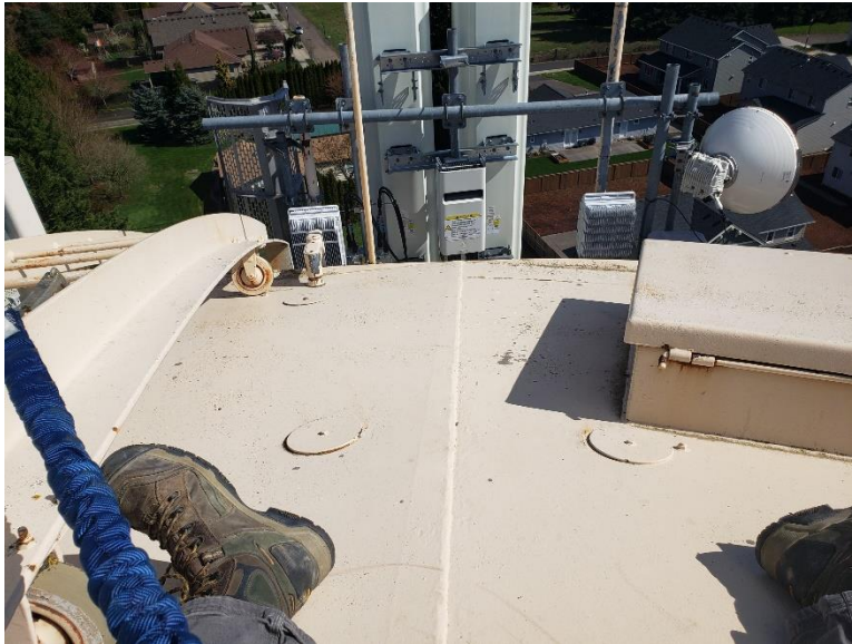
Conduit penetration adjacent ladder at edge.
