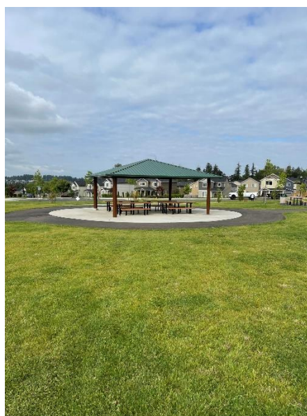
Figure 2: Picnic Structure with picnic tables.
