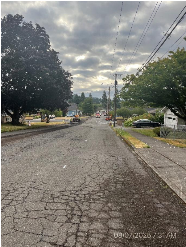
NE 22 ND AVE TRAVEL LANE REPAIRS (BELOW).
