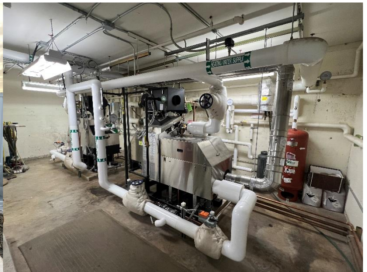
New Chiller (left) and New Boilers (right)
