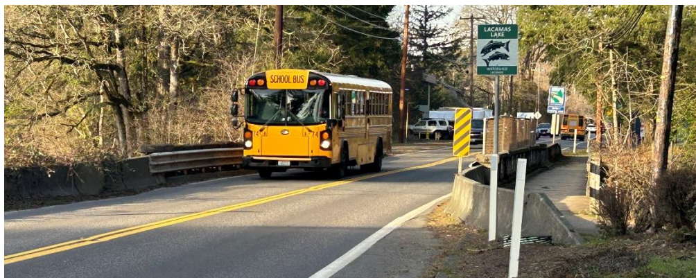
Existing SR500 (Everett Street) Lacamas Lake Bridge
