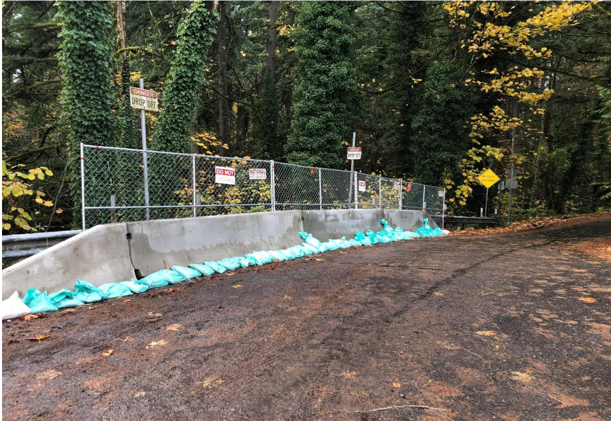
Photo of the Ostenson Canyon Winterization Measures
