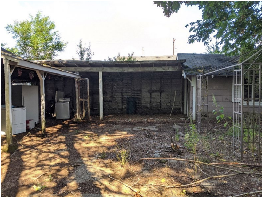
Figure 12. View of outbuildings, facing west.
