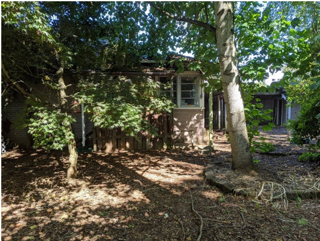
Figure 10. View of single-family residence, facing north.
