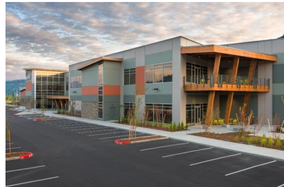
The LEED Silver Insitu Building in Bingen, OR reflects the Pacific Northwest style, including wood siding and drought tolerant landscaping. (Source: lewisbuilds.com/projects/insitu)
