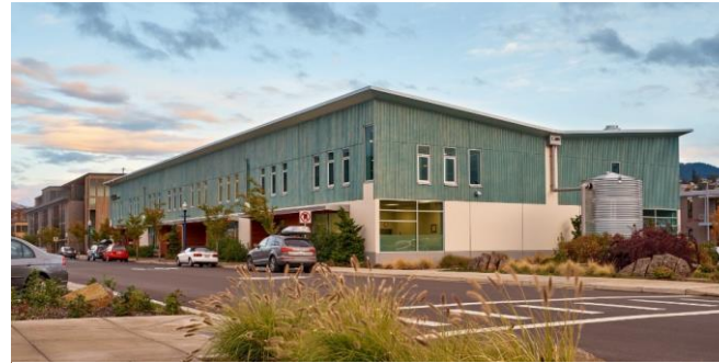
At the LEED Silver Halyard Building in Hood River, OR, rooftop equipment is screened from the street, parking is located behind the building, and a stormwater cistern collects runoff. (Source: Halyard Building 2, robcon.com)
