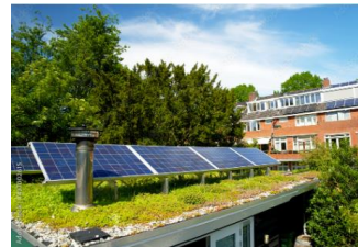
Solar panels on a green roof
