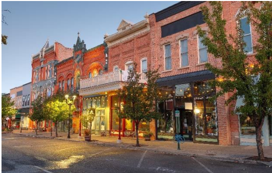
Weather protection and landscaped bollards support a pedestrian friendly streetscape (Source: @ SeanVavonePhoto / Adobe Stock)
