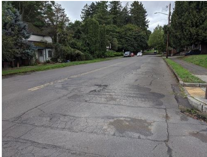
NW 12 th Avenue, looking West from NW Ash Street
