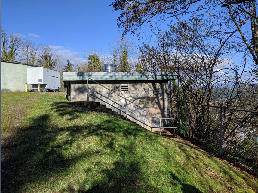
BOOSTER PUMP STATION
