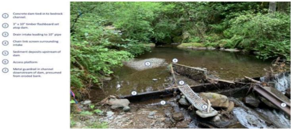
Figure 1: Photo of existing dam and intake structure from downstream of dam looking upstream
