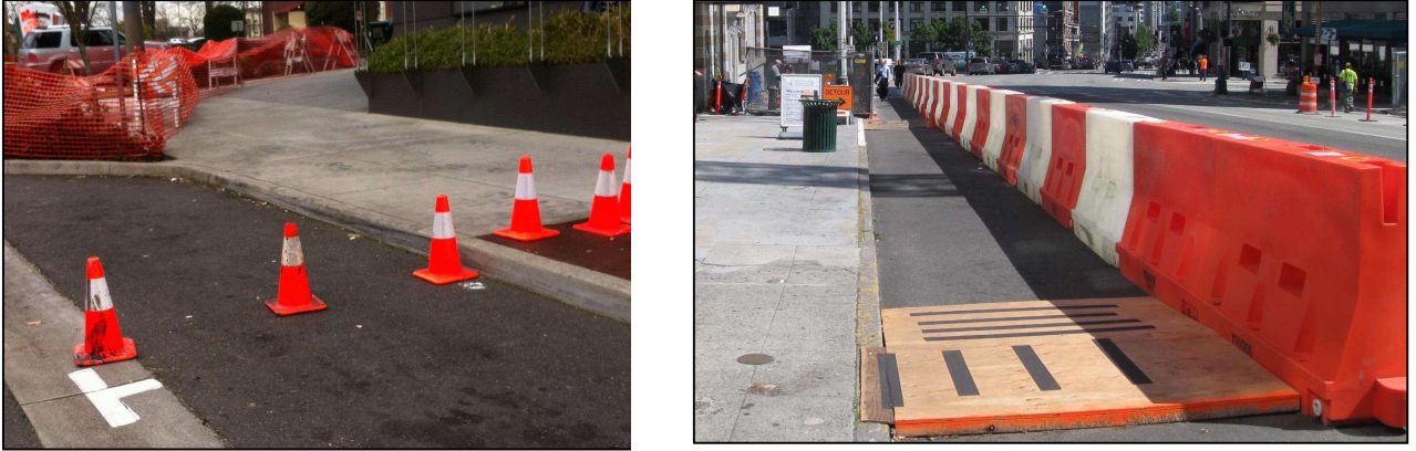
Figure 4: Examples of work zone accessibility, inaccessible versus accessible
