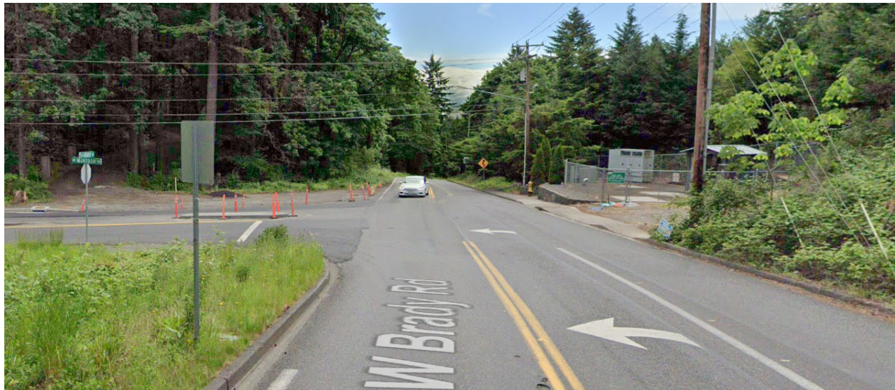
Figure 3- Left-Turn Lane at the Intersection of McIntosh Rd and Brady Rd Provides a Safe Turning Movements
