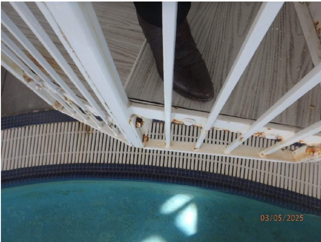
Figure 5: Typical Bolts at Spiral Guardrails
