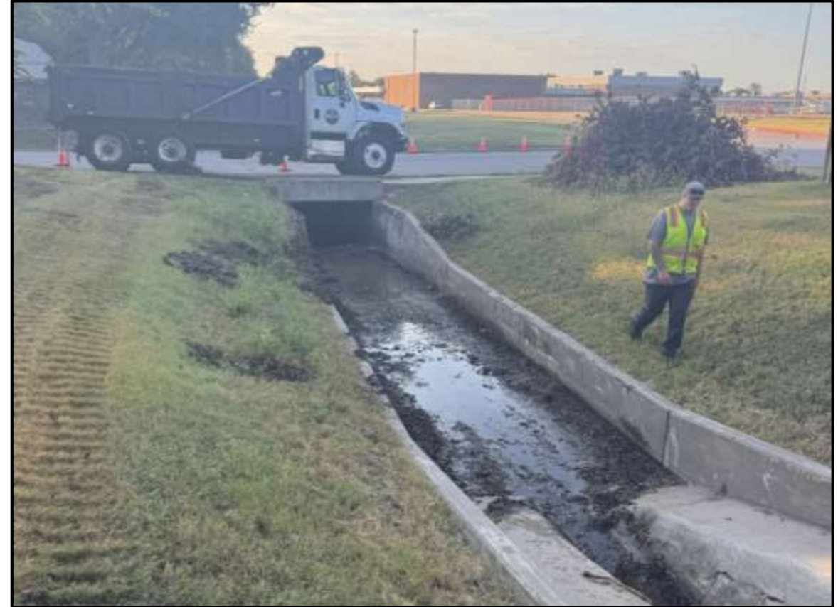
Public Works removed sediment to restore drainage.
