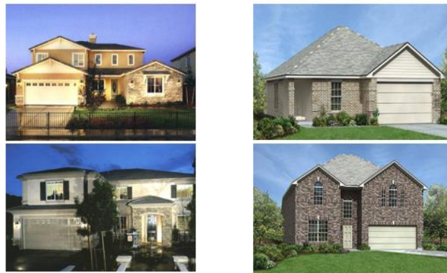
Examples of facades that do not conform to TND requirements.
