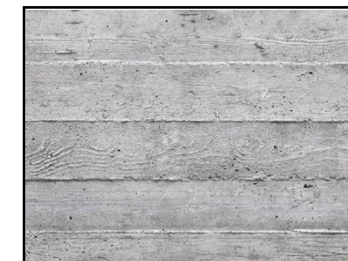
BOARD FORMED CONCRETE- 80 SQ. FT.
