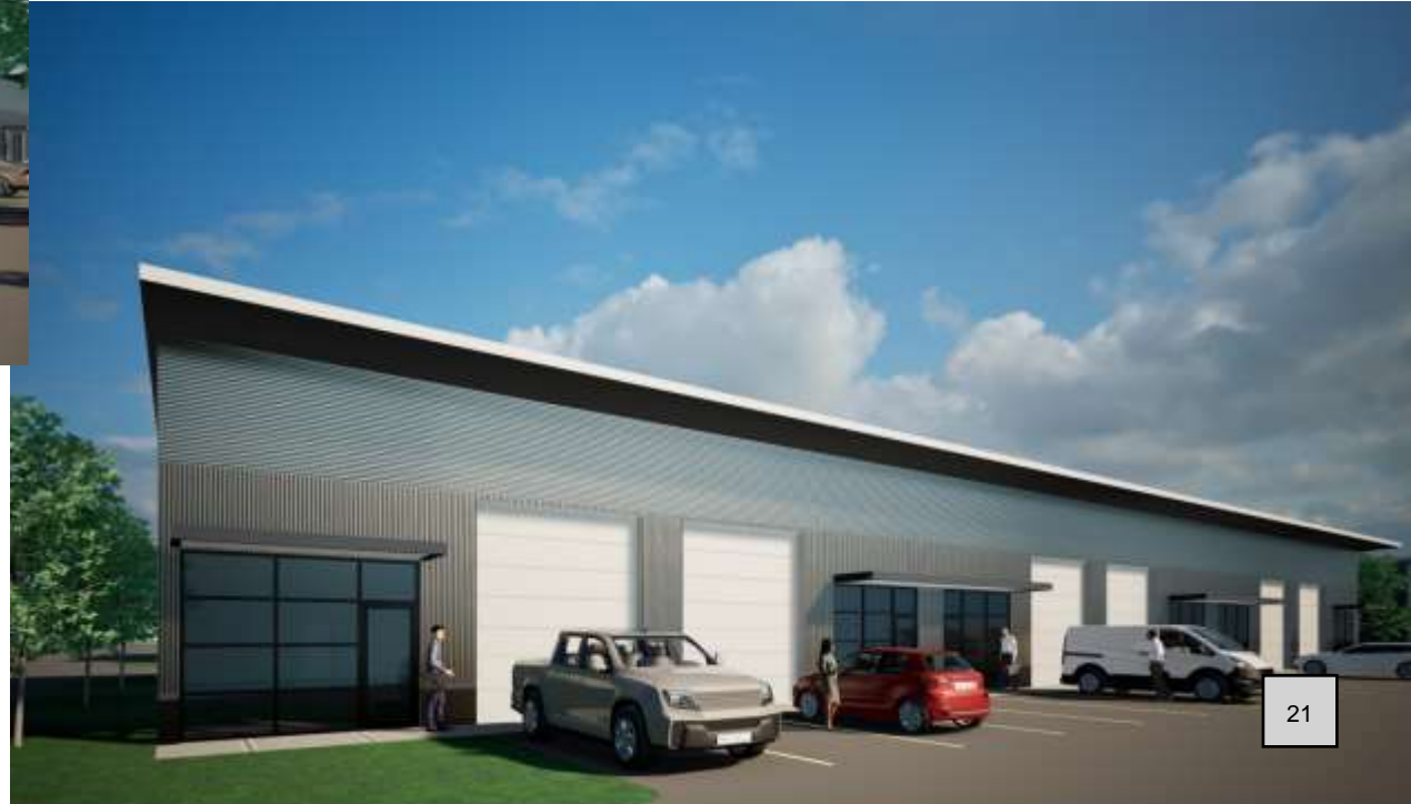
Typical interior to site building
