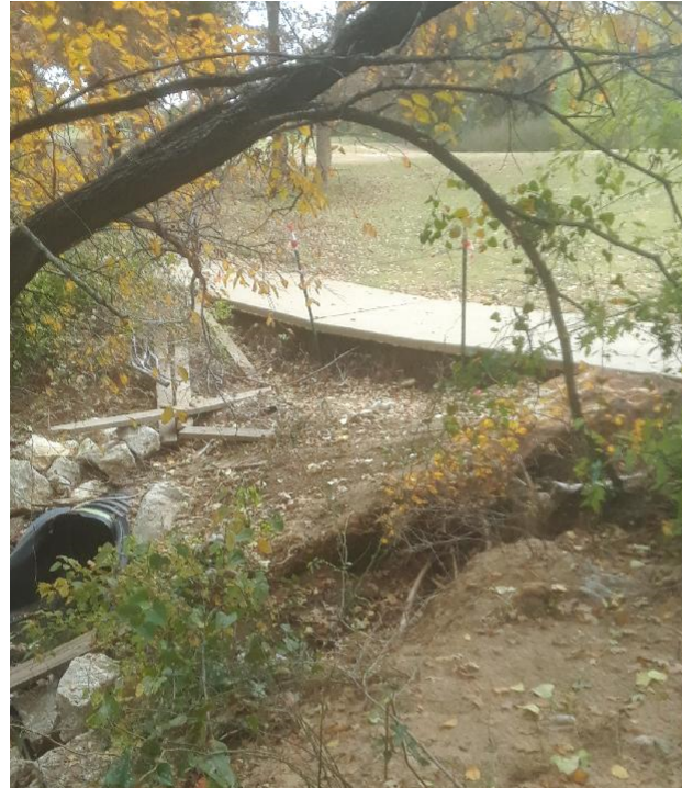
UNDERMINED CART PATH AND DRAINAGE
