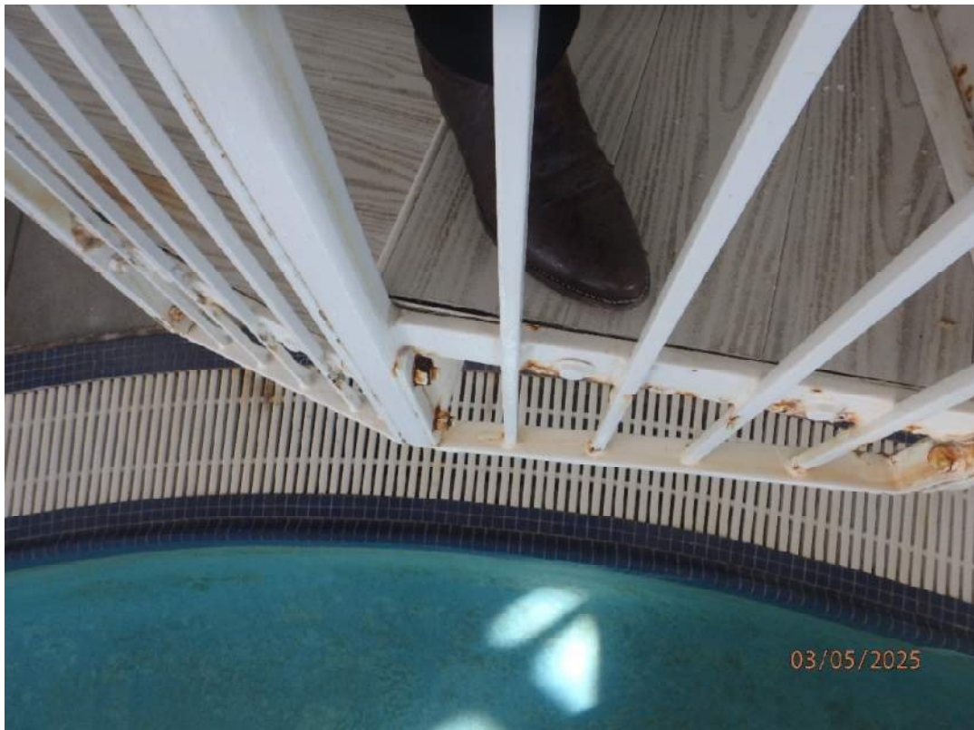
Figure 5: Typical Bolts at Spiral Guardrails
