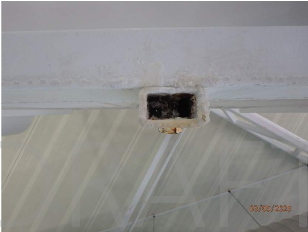
Figure 6: View of Upper Platform Guardrail Bolt – View Inside Post from Below
