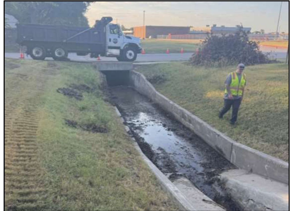
Public Works removed sediment to restore drainage.
