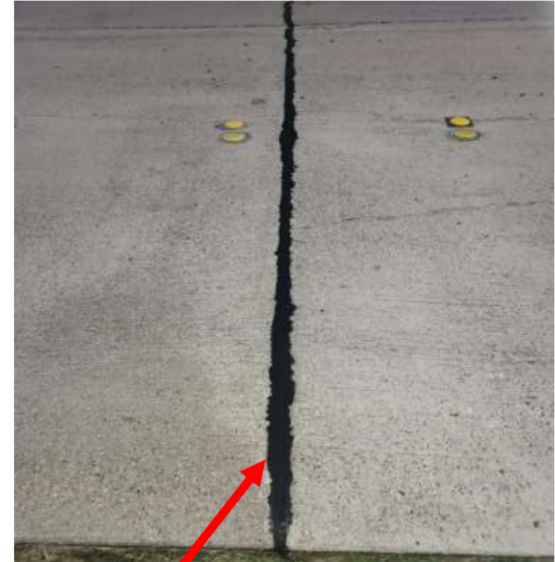
Proper joint seal to prevent water penetration and more costly future repairs
