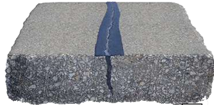
Crack Seal application
