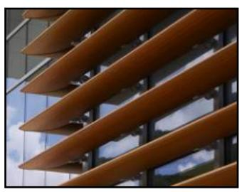
ALUMINUM SHADING DEVICE
