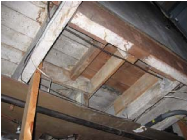
Fig 41: First Floor Structure - Floor infill at previous floor opening east of stair opening
