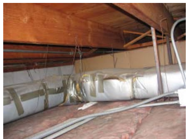
Fig 64: Attic and Roof Structures- Rafters over 1949 addition in good condition
