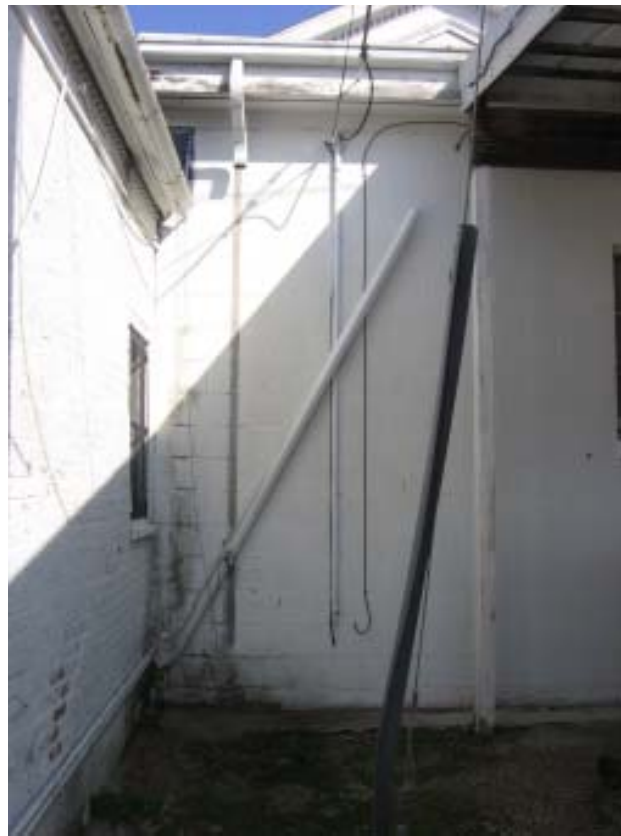
Fig 13: South elevation - Downspouts at corner of 1949 Addition and Jail
