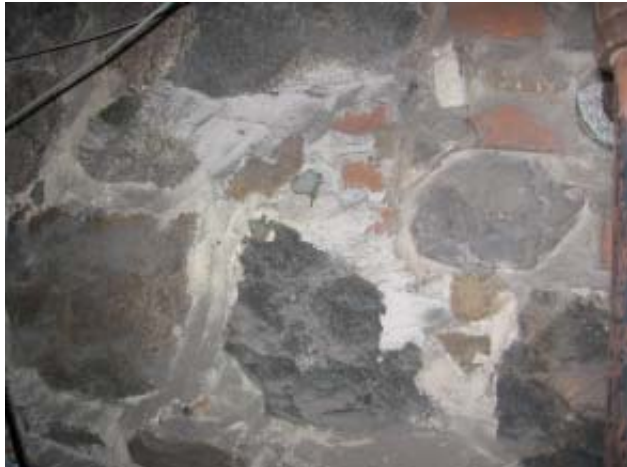
Fig 30: Basement - Cut stone masonry walls repointed
