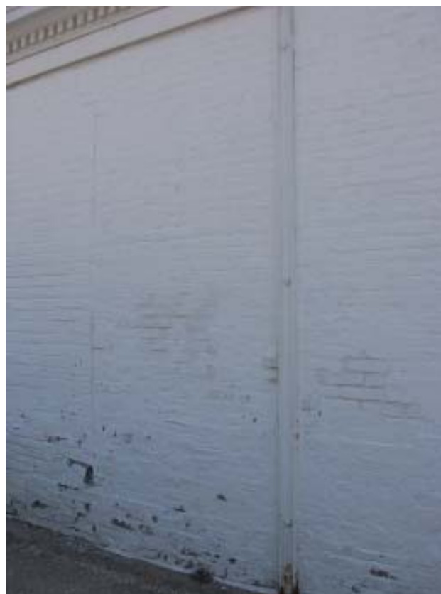
Fig 25: West elevation - Existing channel brace
