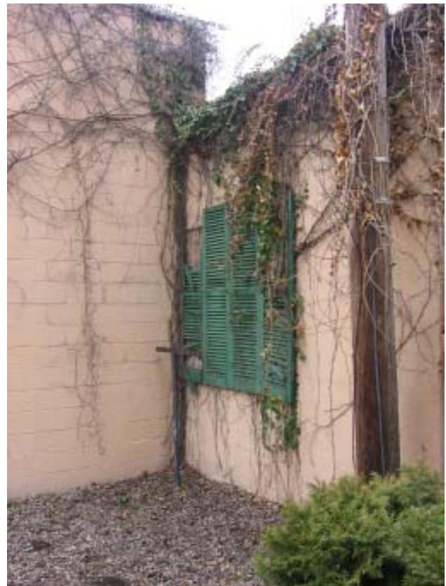
Fig 73: Garage- South elevation, south wall of addition and west wall of original building
