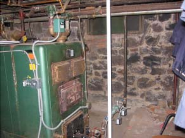
Fig 29: Basement - Cut stone masonry walls
