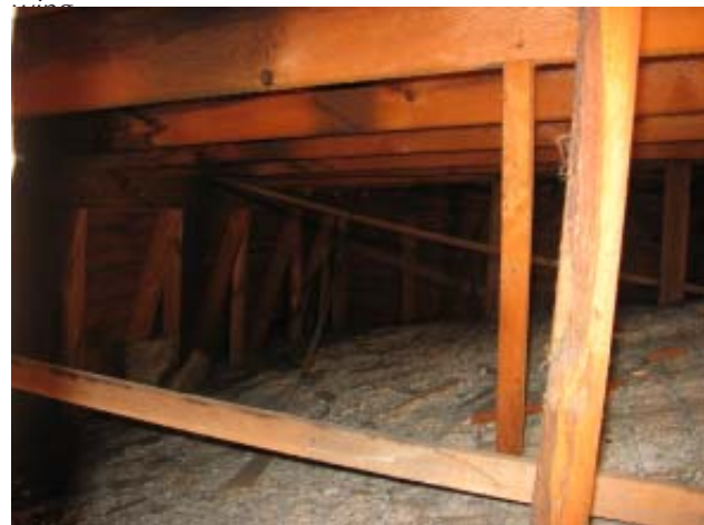
Fig 58: Attic and Roof Structures- Bracing of mansard roof construction of west wing
