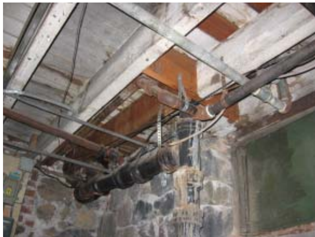
Fig 40: First Floor Structure - Floor infill at previous floor opening in southeastern corner
