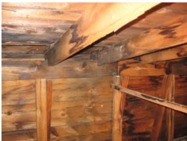
Fig 59: Attic and Roof Structures- Mansard roof construction details, note water staining in wood members in west wing
