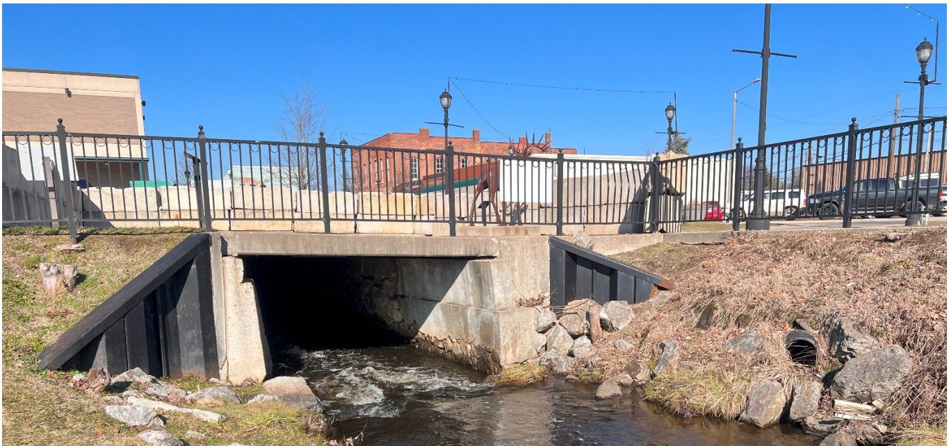
Figure 1: Image of failing culvert parallel to Days Avenue facing north (Buchanan, MI). Note: failure area inside culvert is approximately 10-20' into the culvert.
