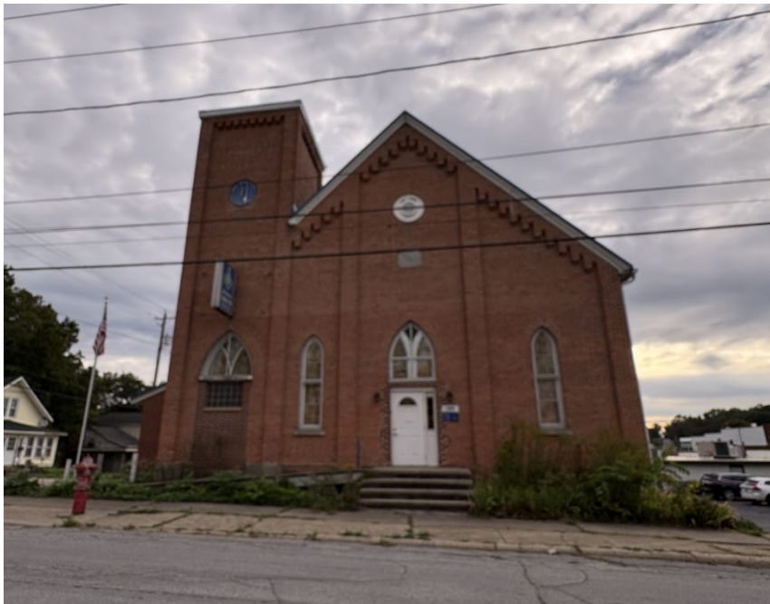
New roof view from N Oak Street looking east.
