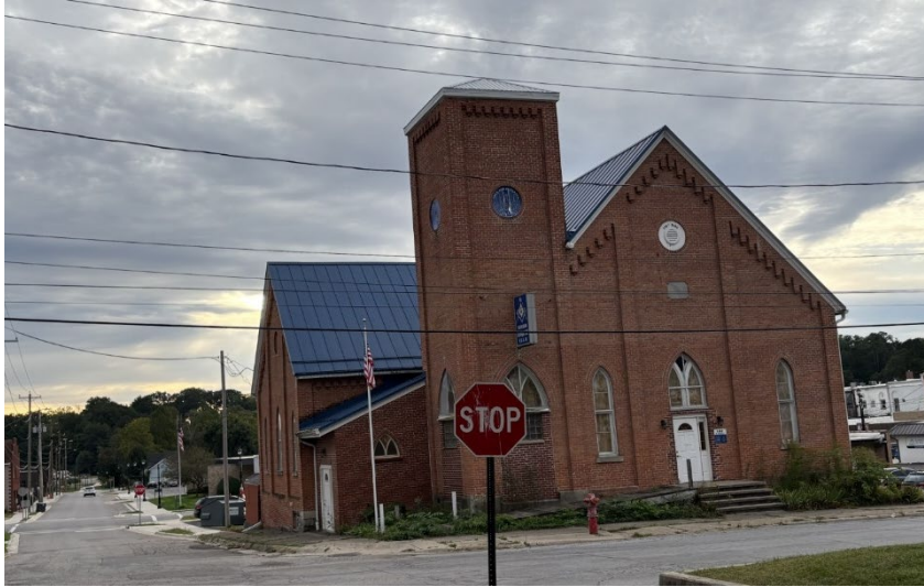
New roof view from W Dewey Street
