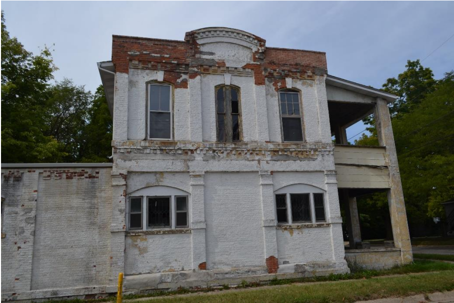
Zinc Collar Pad Building, 304 S. Oak (2009)
