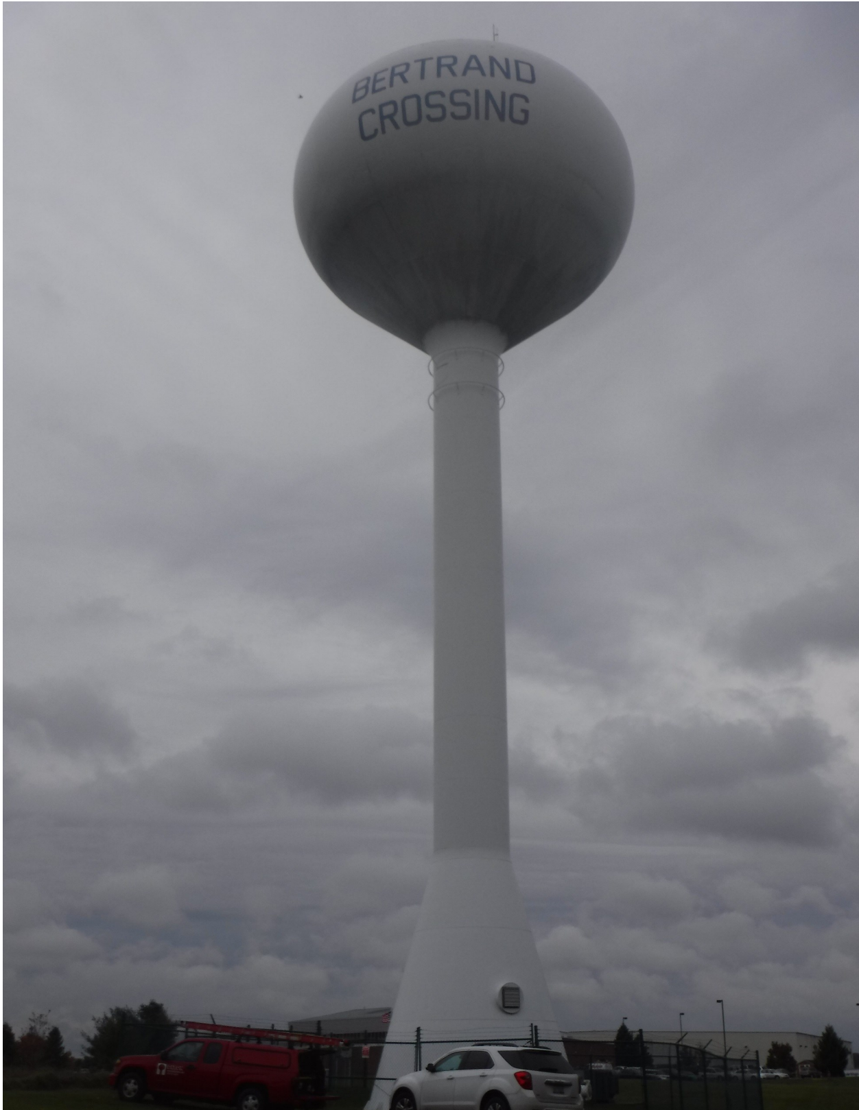
300,000 gallon spheroid owned by Bertrand Township.
