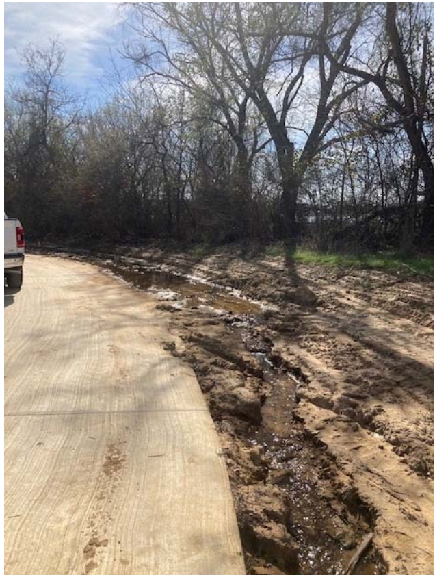
March 7, 2023 -Drainage coming from adjacent resevoir to the south of the development overflows into the ditch on the south side of the development. This was overlooked in the development design as the natural flow came from a pipe that extended into the property. That pipe was removed and water diverted into the ditches. This has created erosion as well as standing water in various locations.
