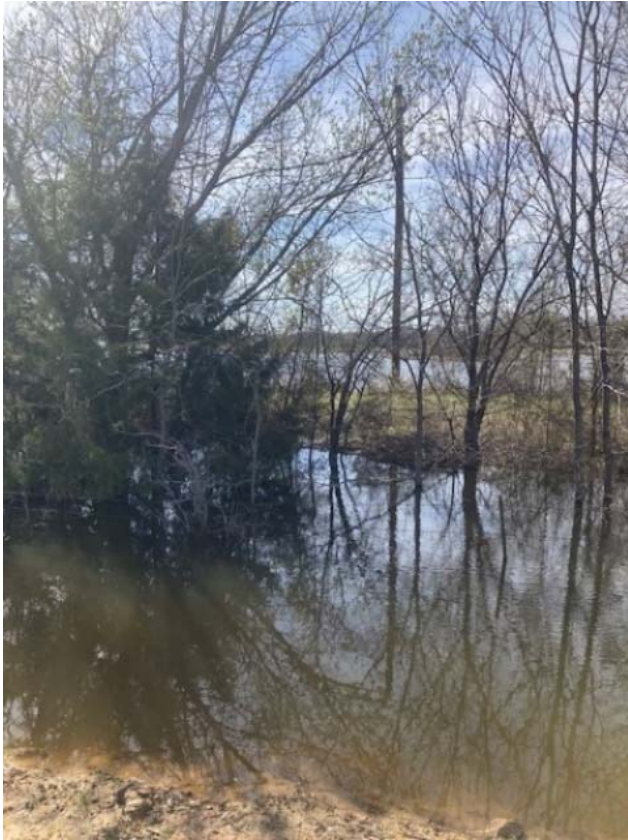
March 7, 2023 -Drainage coming from adjacent resevoir to the south of the development overflows into the ditch on the south side of the development. This was overlooked in the development design as the natural flow came from a pipe that extended into the property. That pipe was removed and water diverted into the ditches. This has created erosion as well as standing water in various locations.
