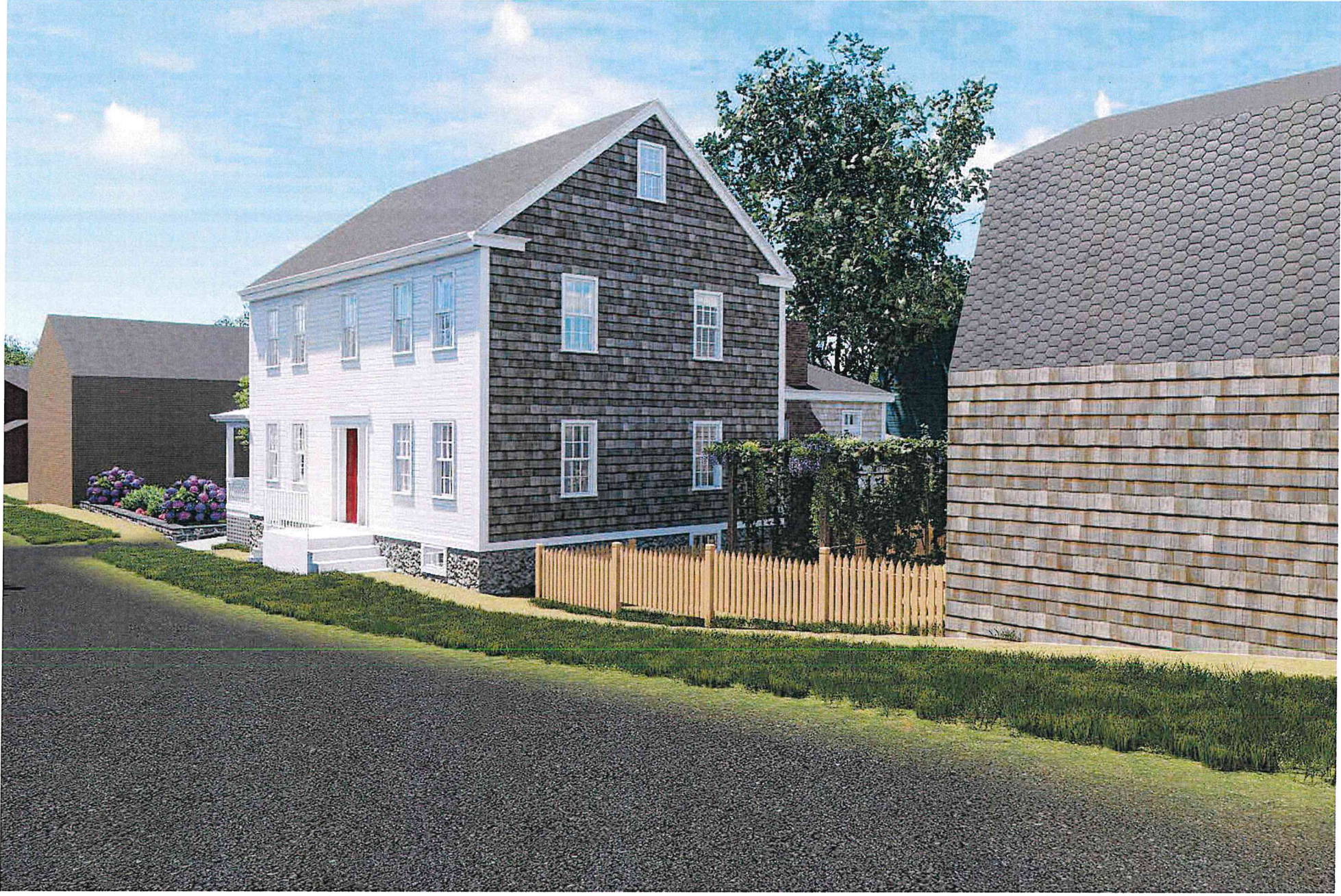
FRONT EAST SIDE VIEW
