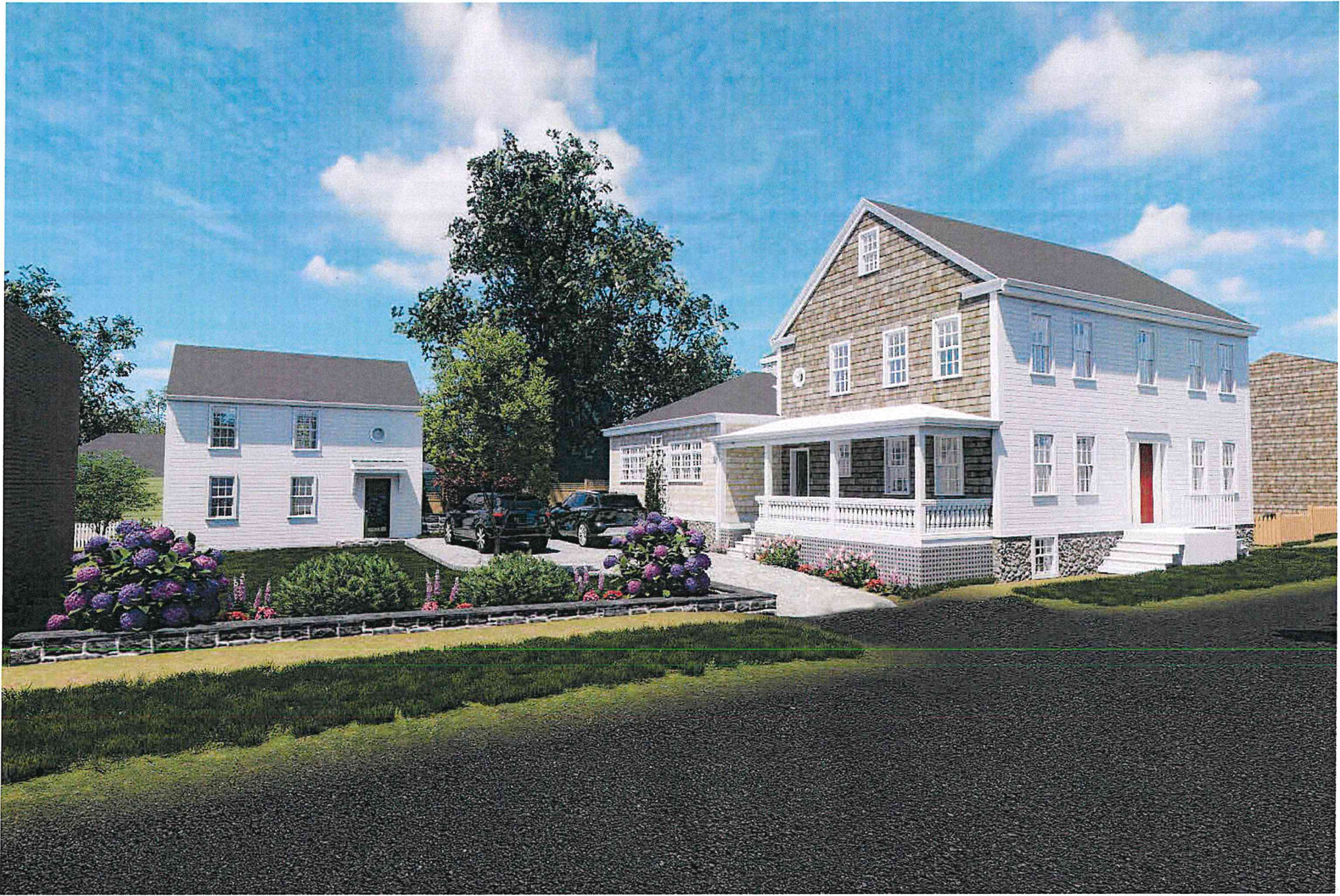
FRONT WEST SIDE VIEW
