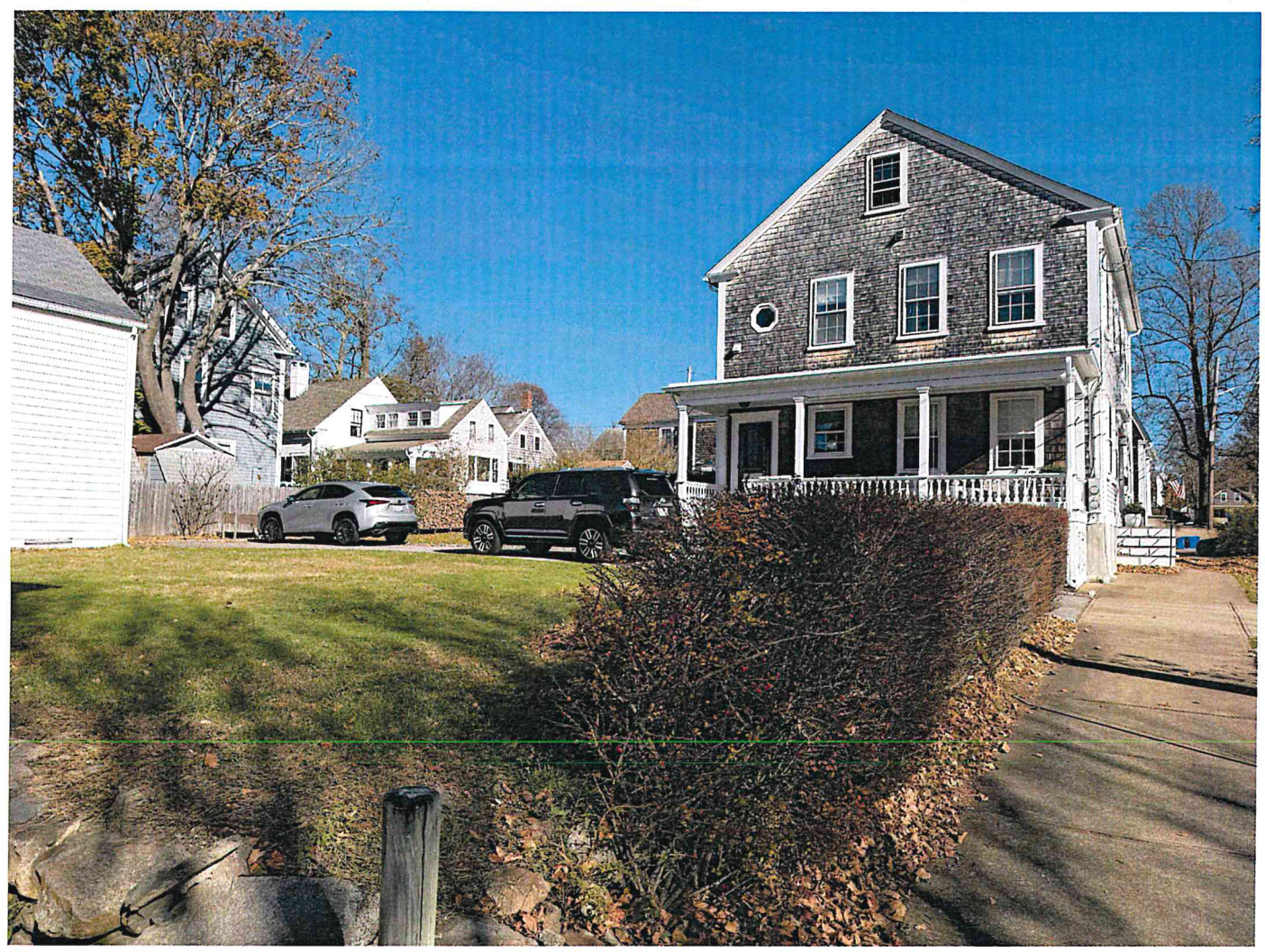
Photo #1: Front West side view, southwest corner of property
