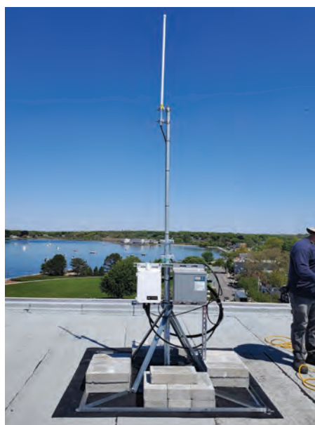
Antennae for new smart meter system.
