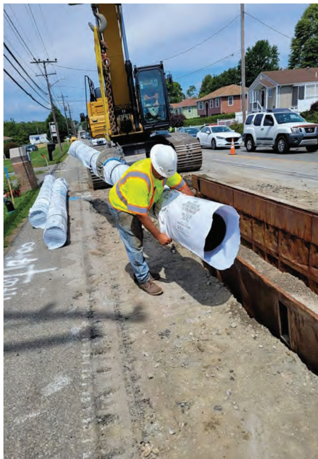
A new 12-inch main is installed on Metacom Ave. in Bristol.
