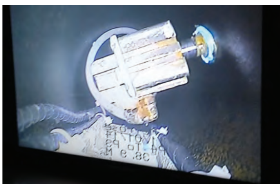
Old cast iron pipe before cleaning and lining.
