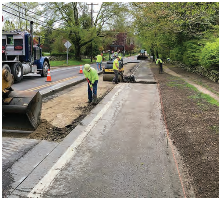
Paving the road after water main installation.
