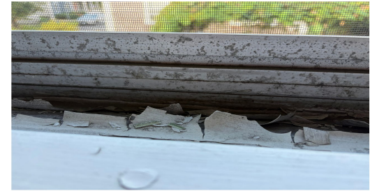
Window #5 Bathroom interior
