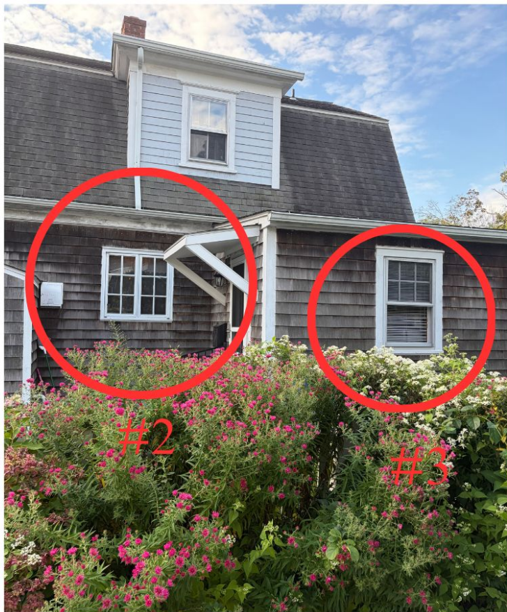
Window #3 Back Porch exterior
