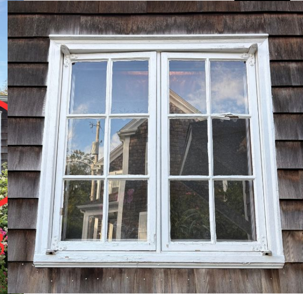
Window #2 Double Hung Kitchen exterior
