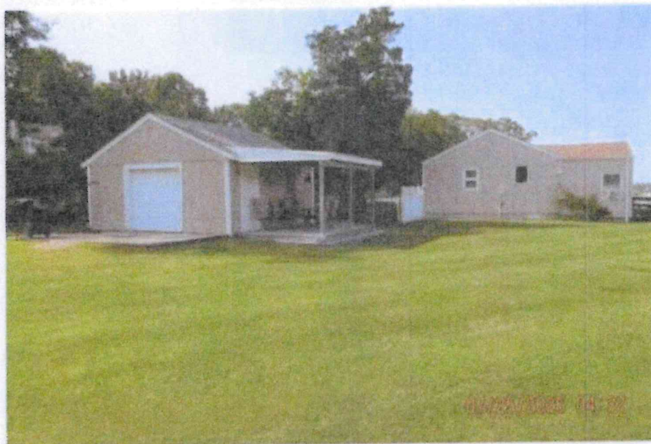
Cottage & Garage - to be demolished
