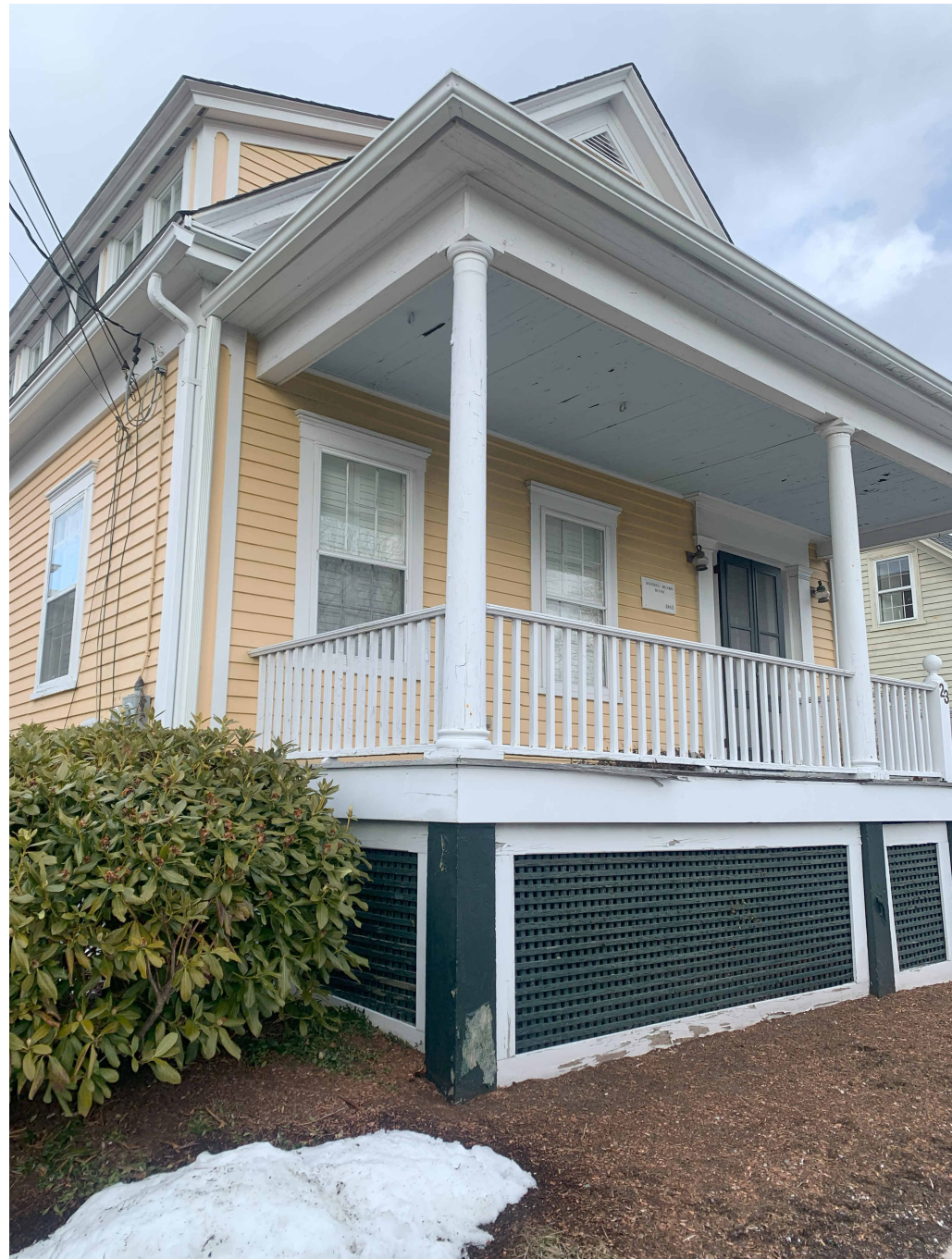
Photo #6: View of southwest corner of front porch
