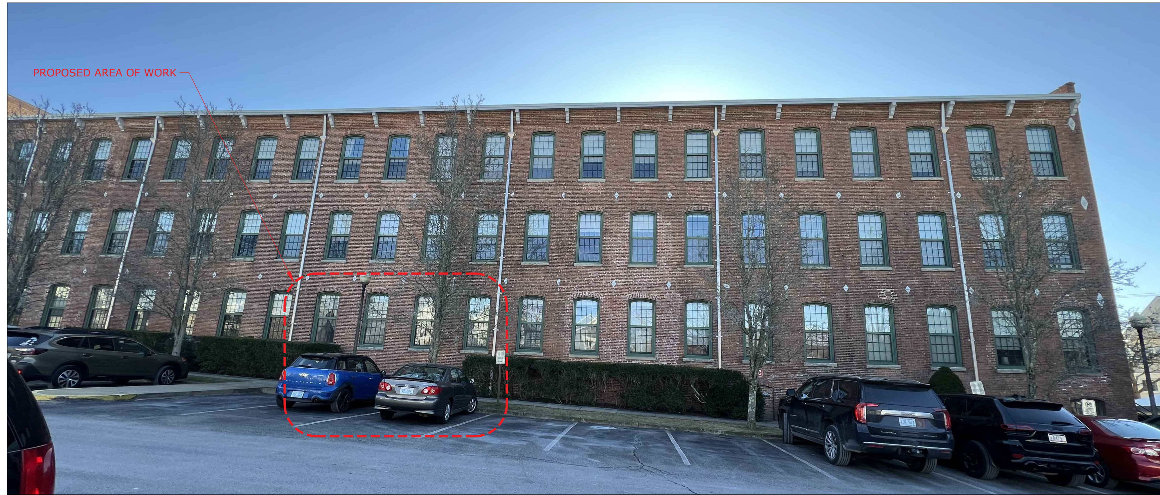
1 NORTH ELEVATION PHOTOGRAPH
