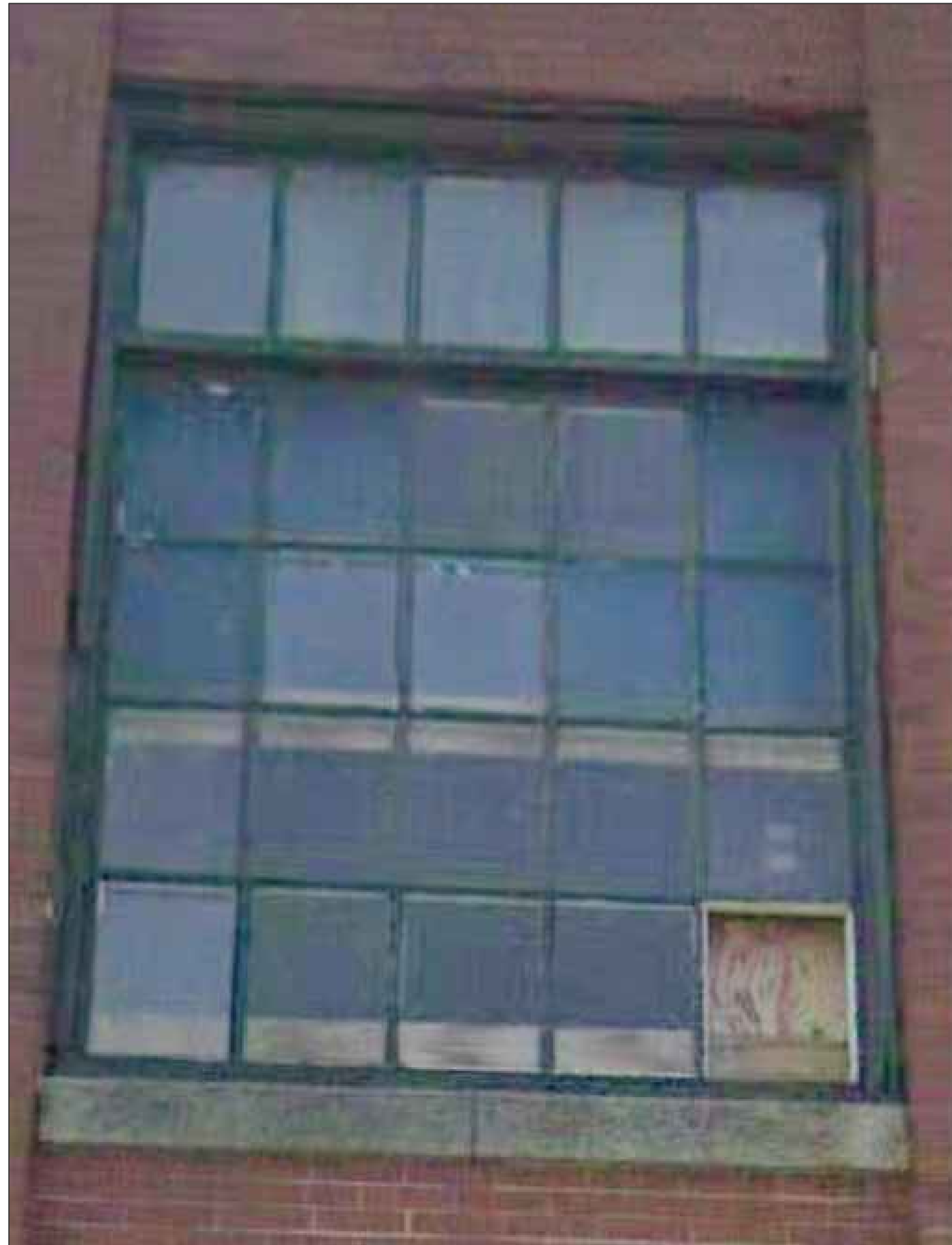
Building 7A Original Wooden Window Exterior
