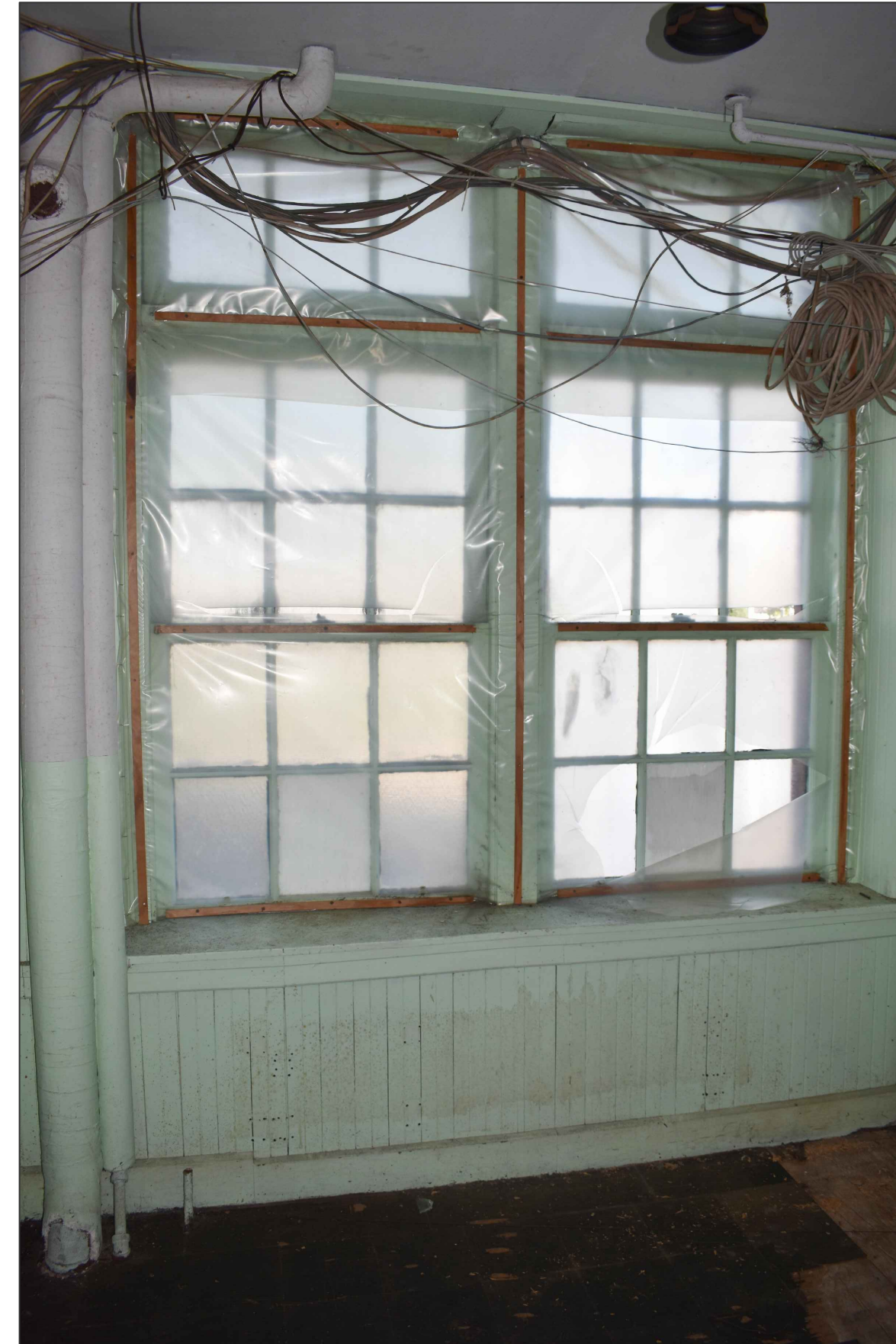
Building 4 Original Wooden Window Interior
