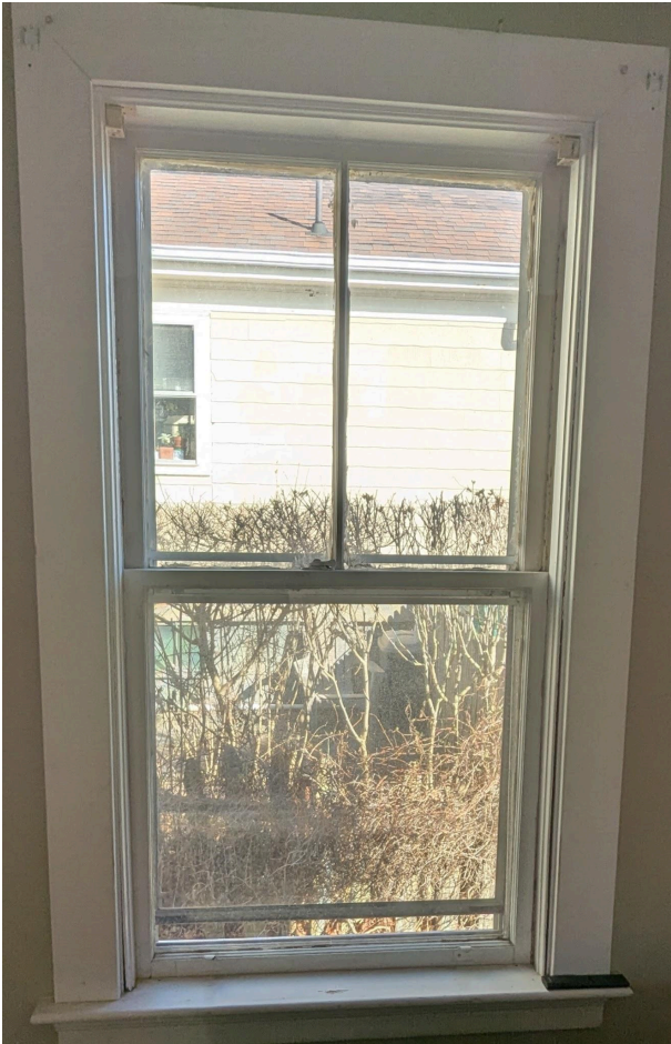
2-over-1 window (east elevation)
