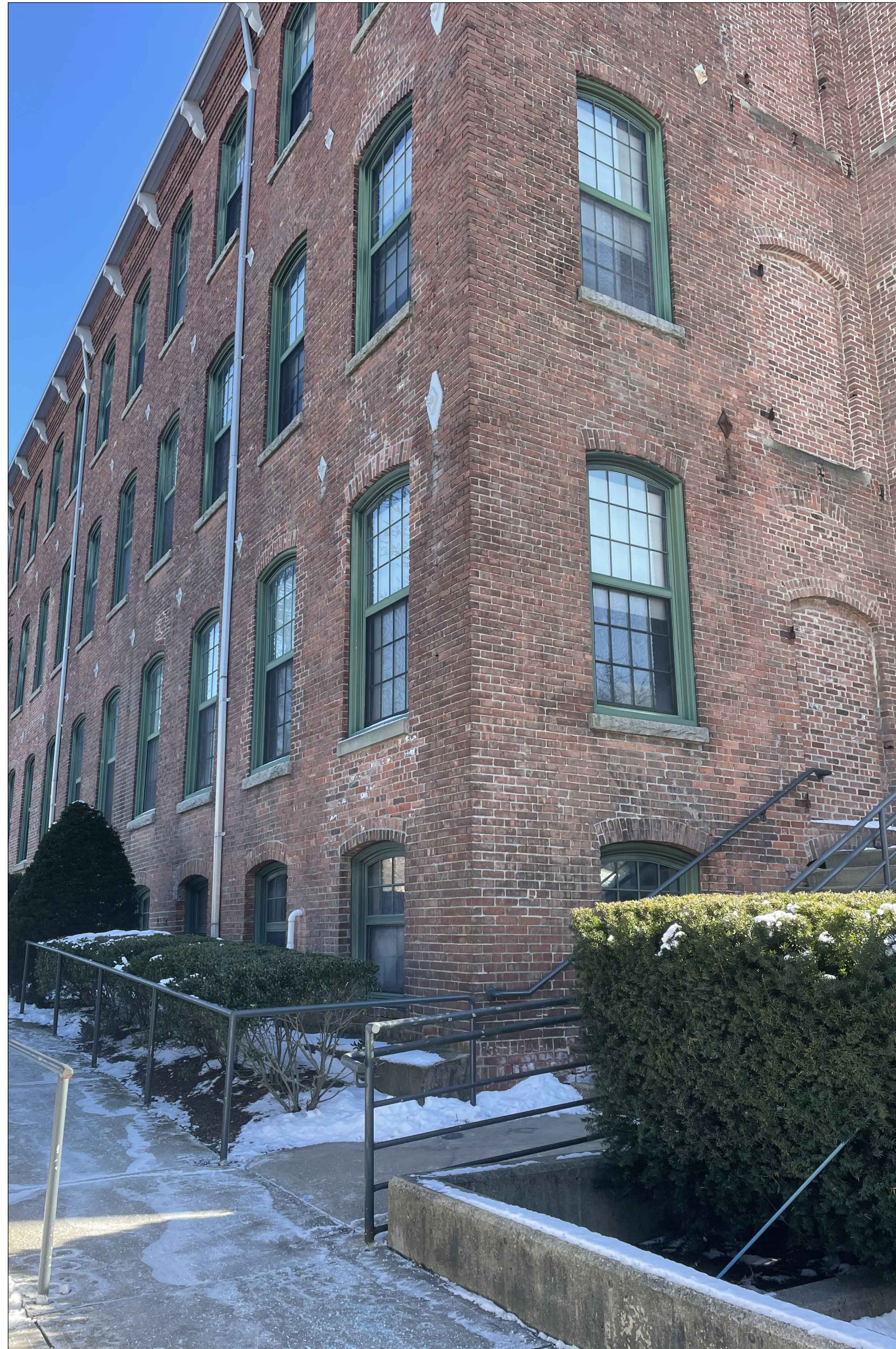
① NORTHWEST ELEVATION PHOTOGRAPH
