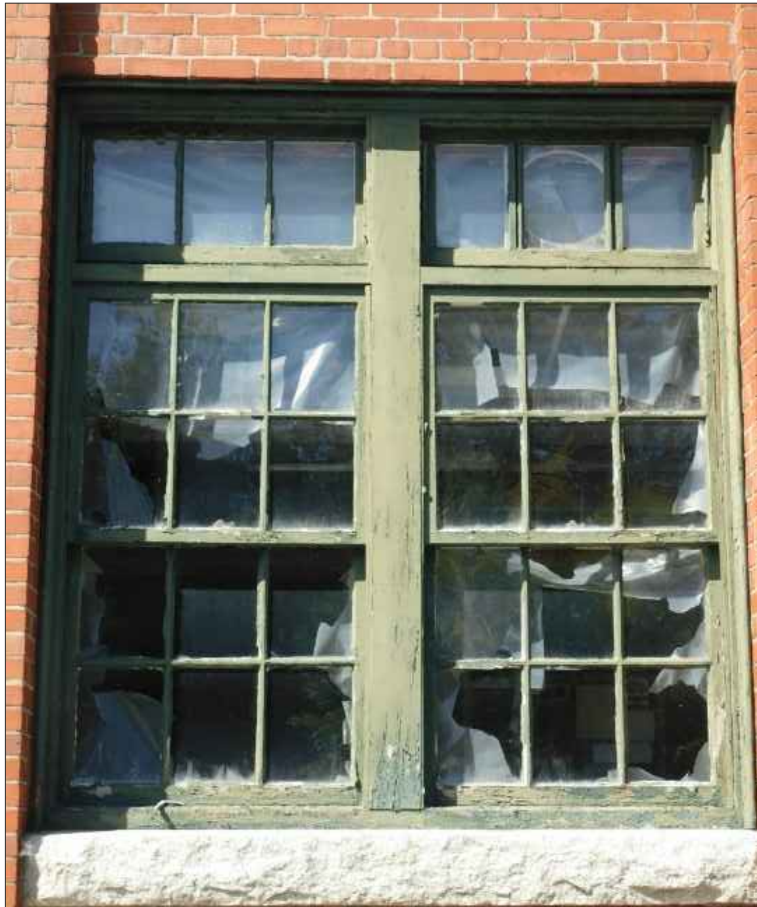
Building 4 Original Wooden Window Exterior
