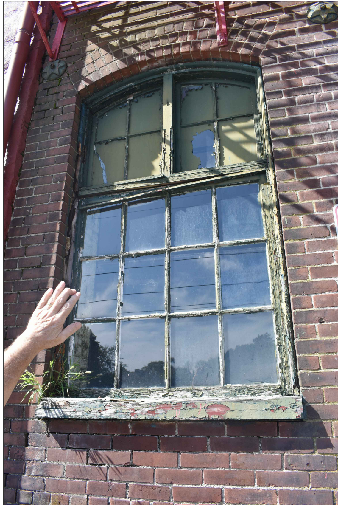
Building 3 Original Wooden Window Exterior
