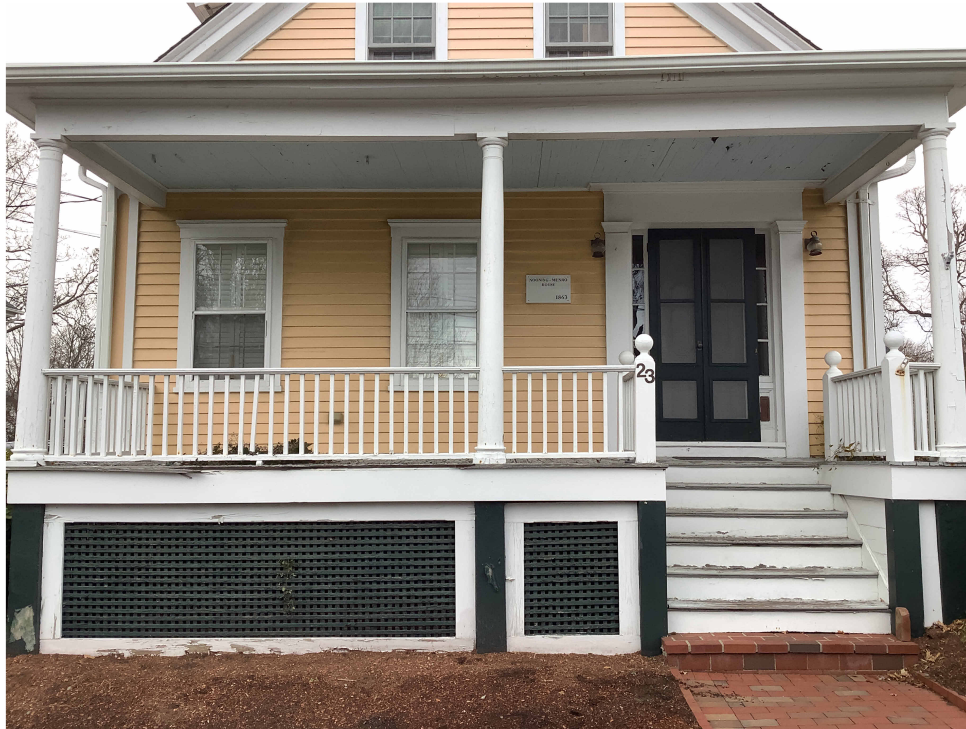
Photo #5: Front view of existing porch
