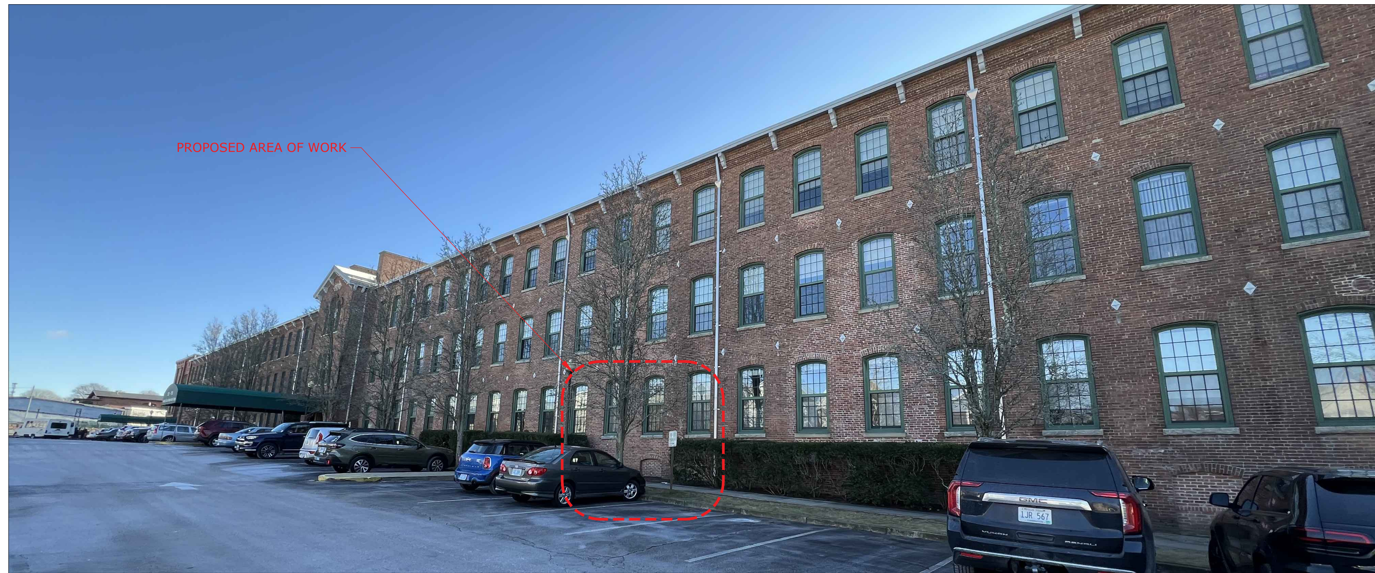
2 NORTHEAST ELEVATION PHOTOGRAPH
