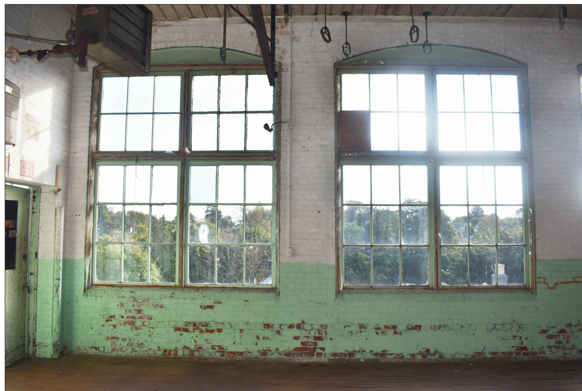
Building 7 Original Wooden Window Interior
