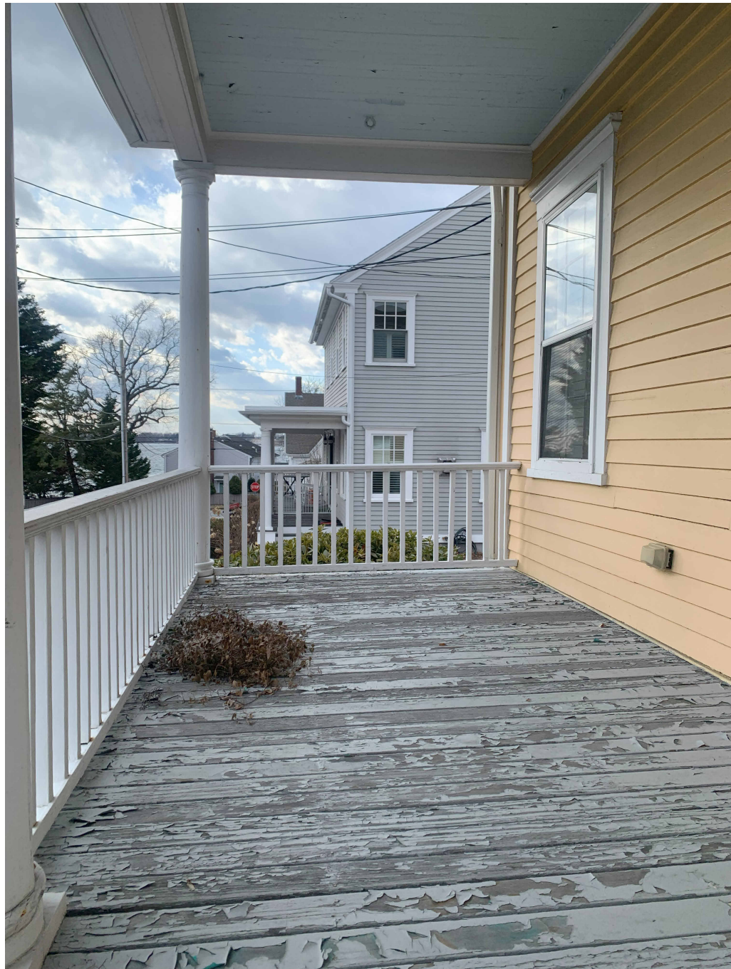
Photo #8: View of existing front porch decking
