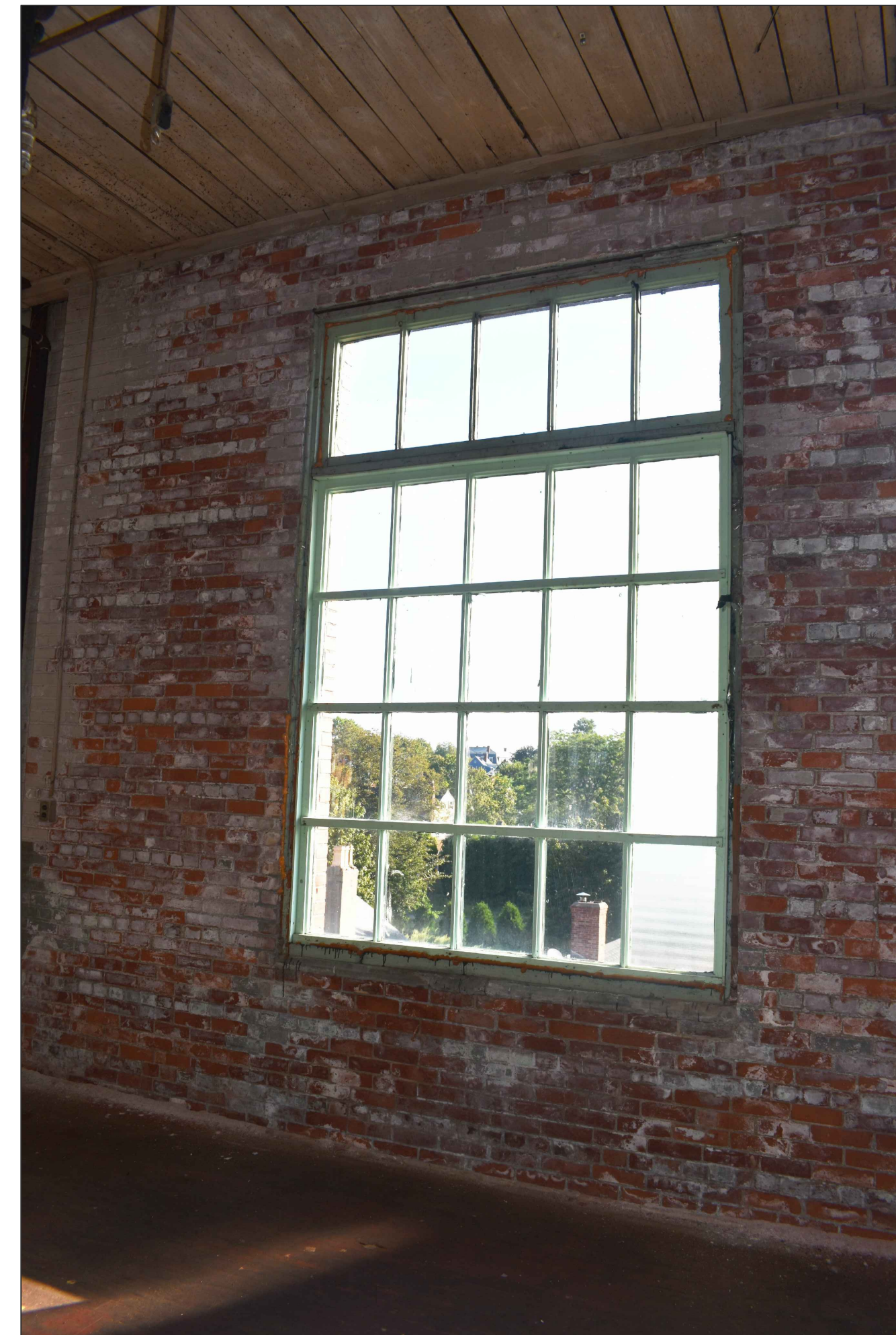
Building 7A Original Wooden Window Interior
