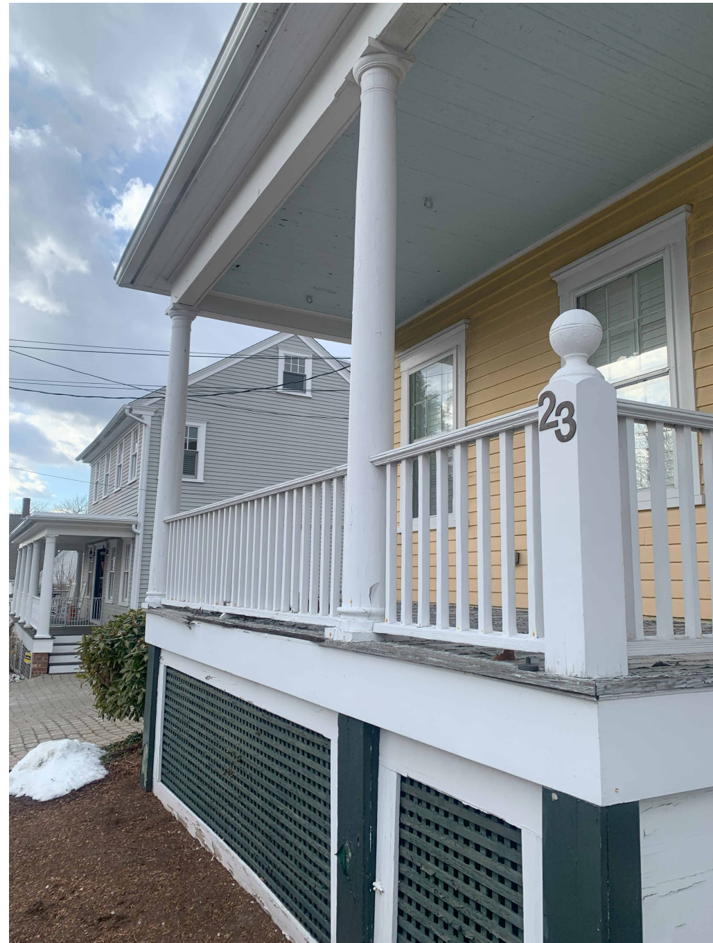
Photo #7: View of southeast corner of front porch
