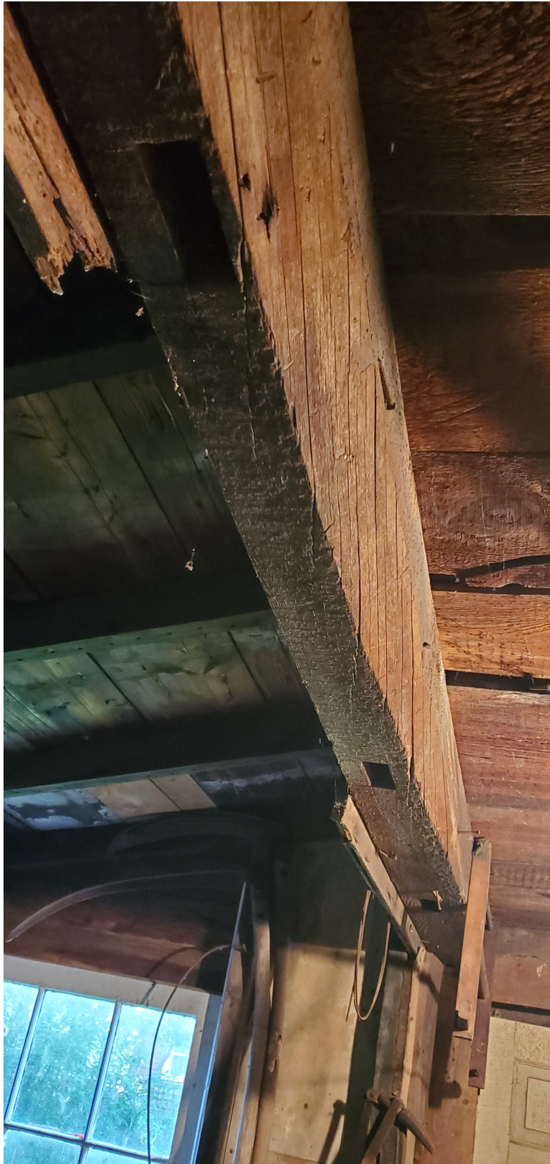
Figure 8: Rear wall showing the beam pockets where framing timbers were removed when building was lengthened in the early 1900s
