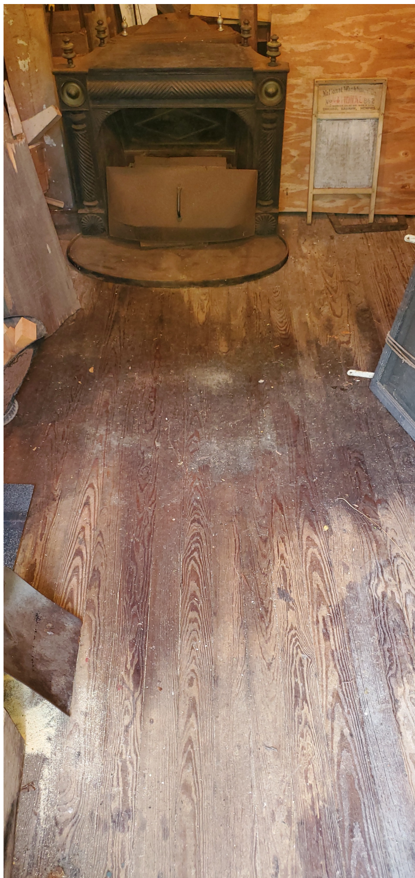
Figure 3: Carriage House first floor hard-wood floor boards
