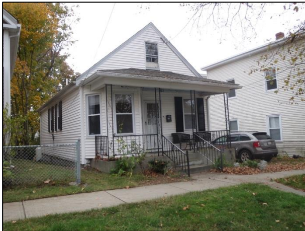
Left: 115 Union Street - Porch replaced with concrete deck and iron posts and railings.
