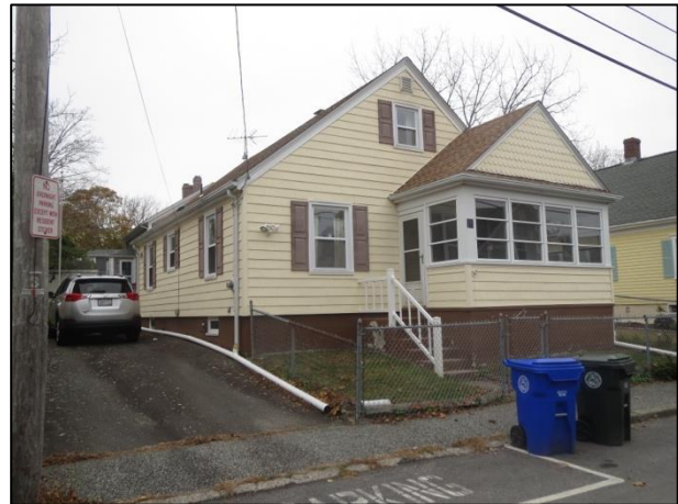
Left: 115 Union Street - Porch replaced with concrete deck and iron posts and railings.
