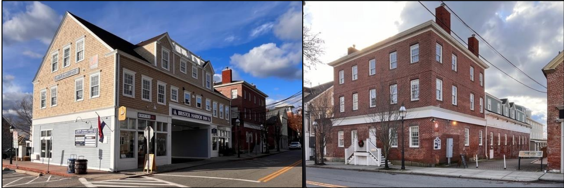
Left: 251 Thames Street, built c. 2004.
