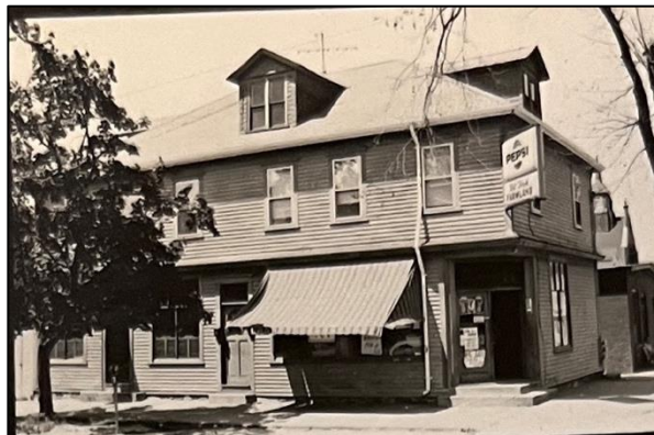
125-129 Franklin Street, September 1972
