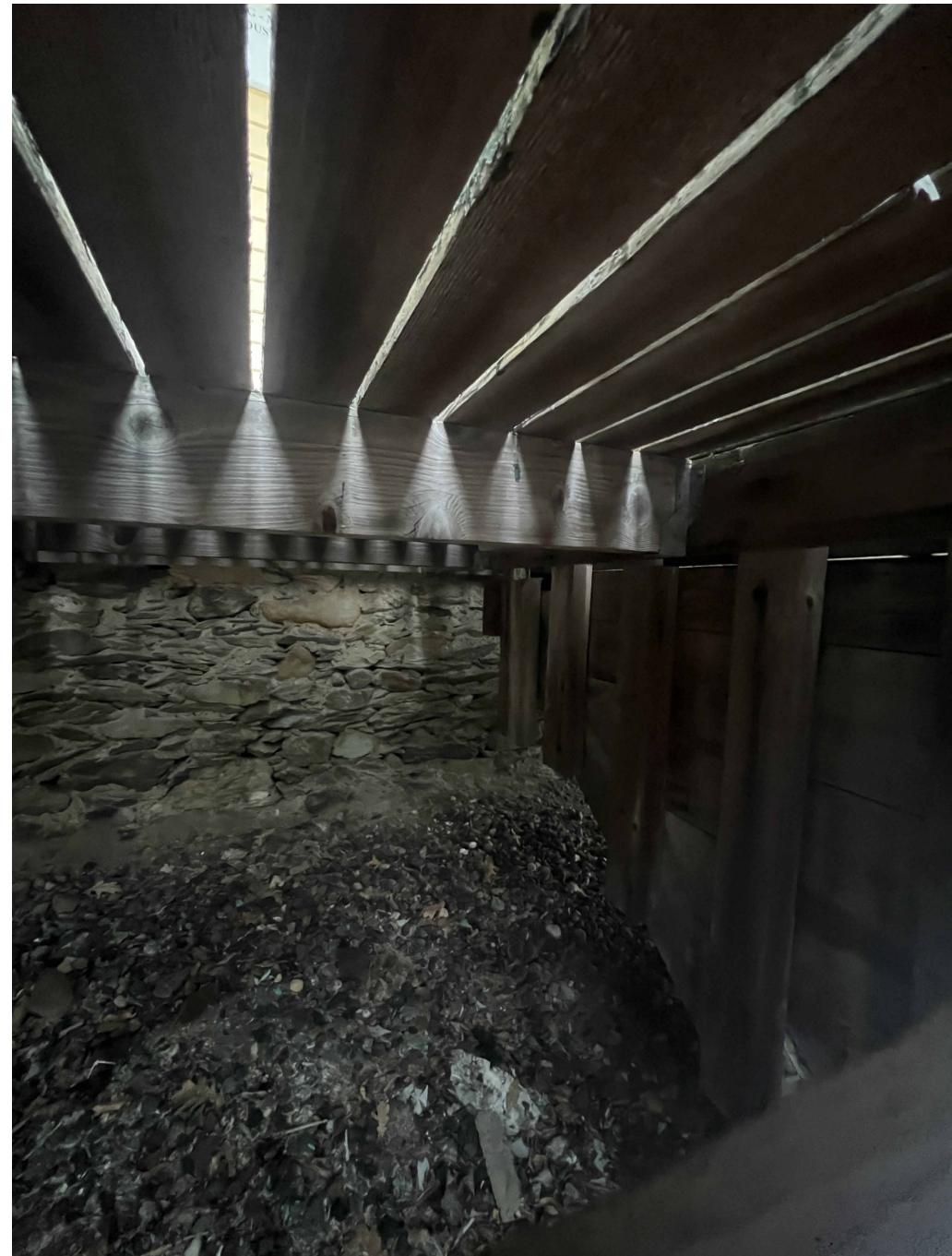
Photo #9: View of existing structure below front porch
