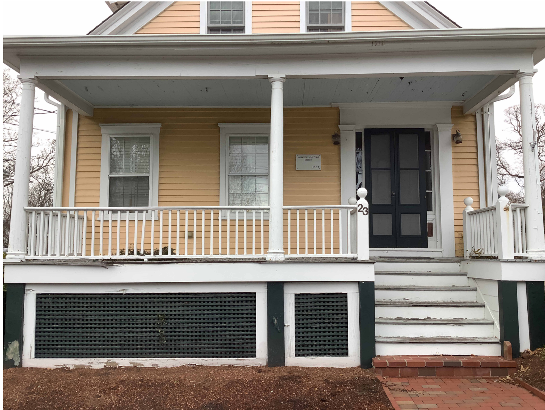
Photo #5: Front view of existing porch
