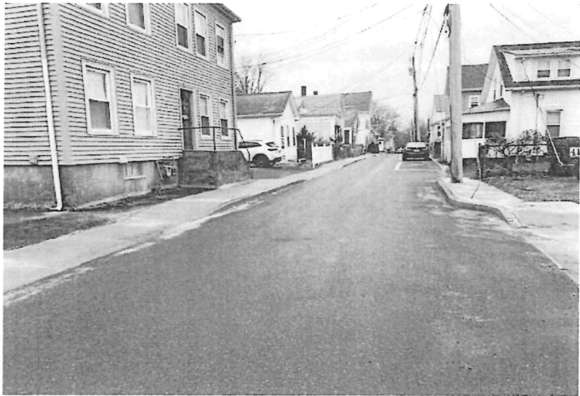
45 Congregational Street- westbound view 14' 6" curb to curb
