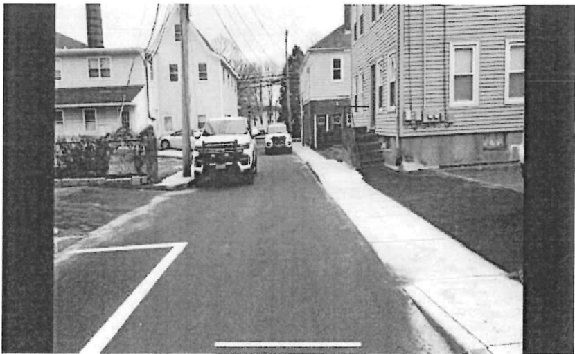
45 Congregational Street- eastbound view with parked vehicle.
