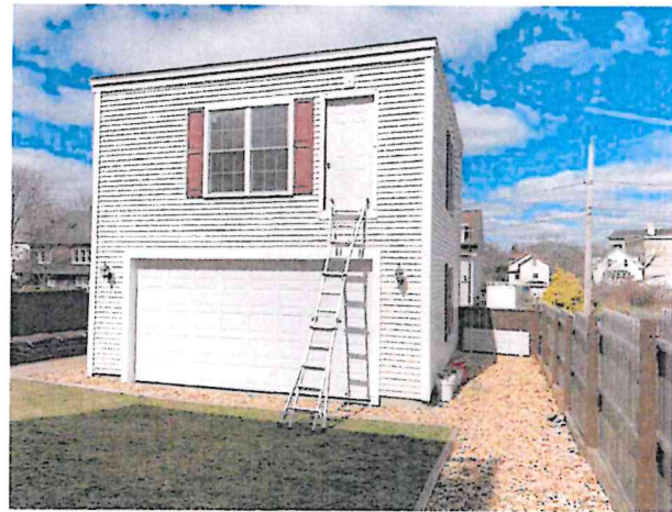
Current Ladder Access
