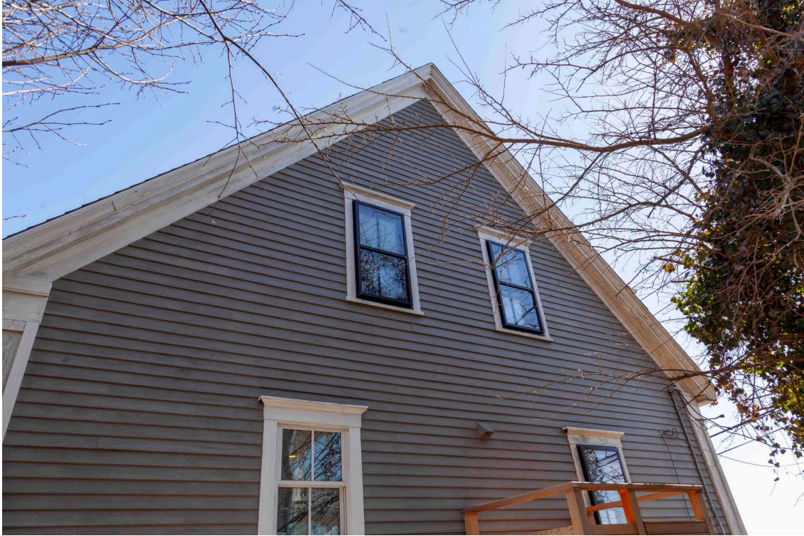
Photo 7 - Existing Wall to have New Window Installed Under Roof Ridge
