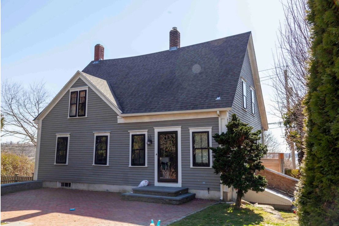
Photo 3 - North View of the Existing Residence
