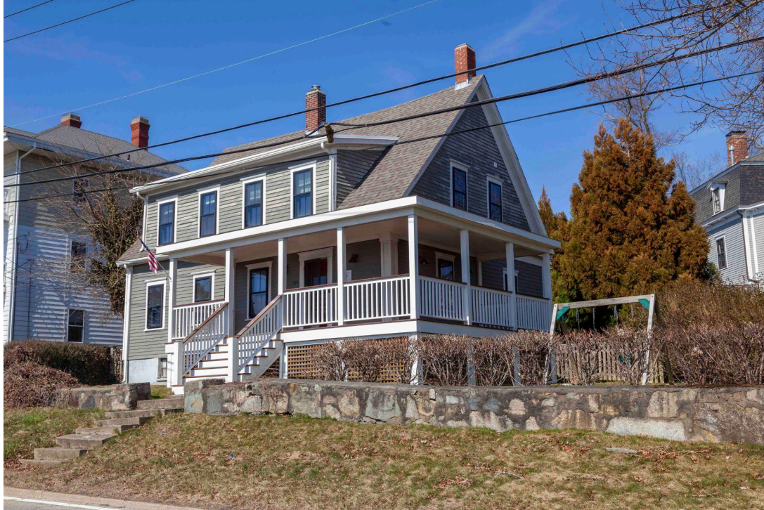
Photo 1 - South View of the Existing Residence
