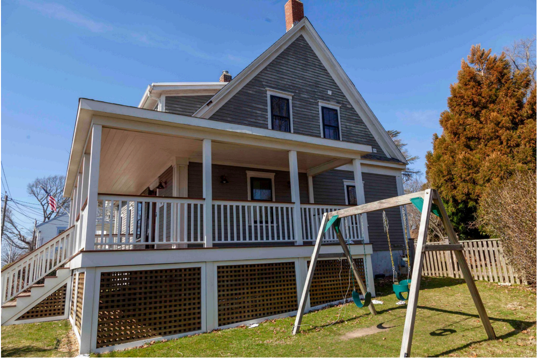
Photo 4 - Southeast View of the Existing Residence
