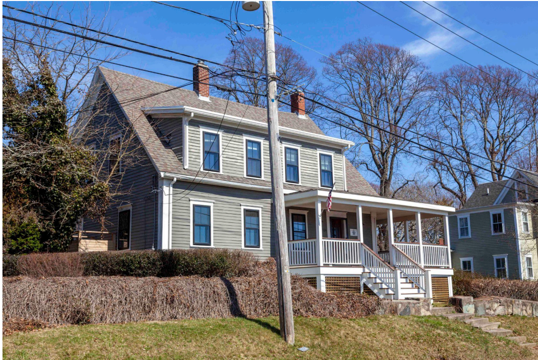
Photo 2 - West View of the Existing Residence
