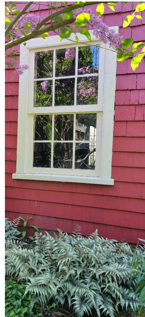
Photo #7: North double-hung 6-over-6 window
