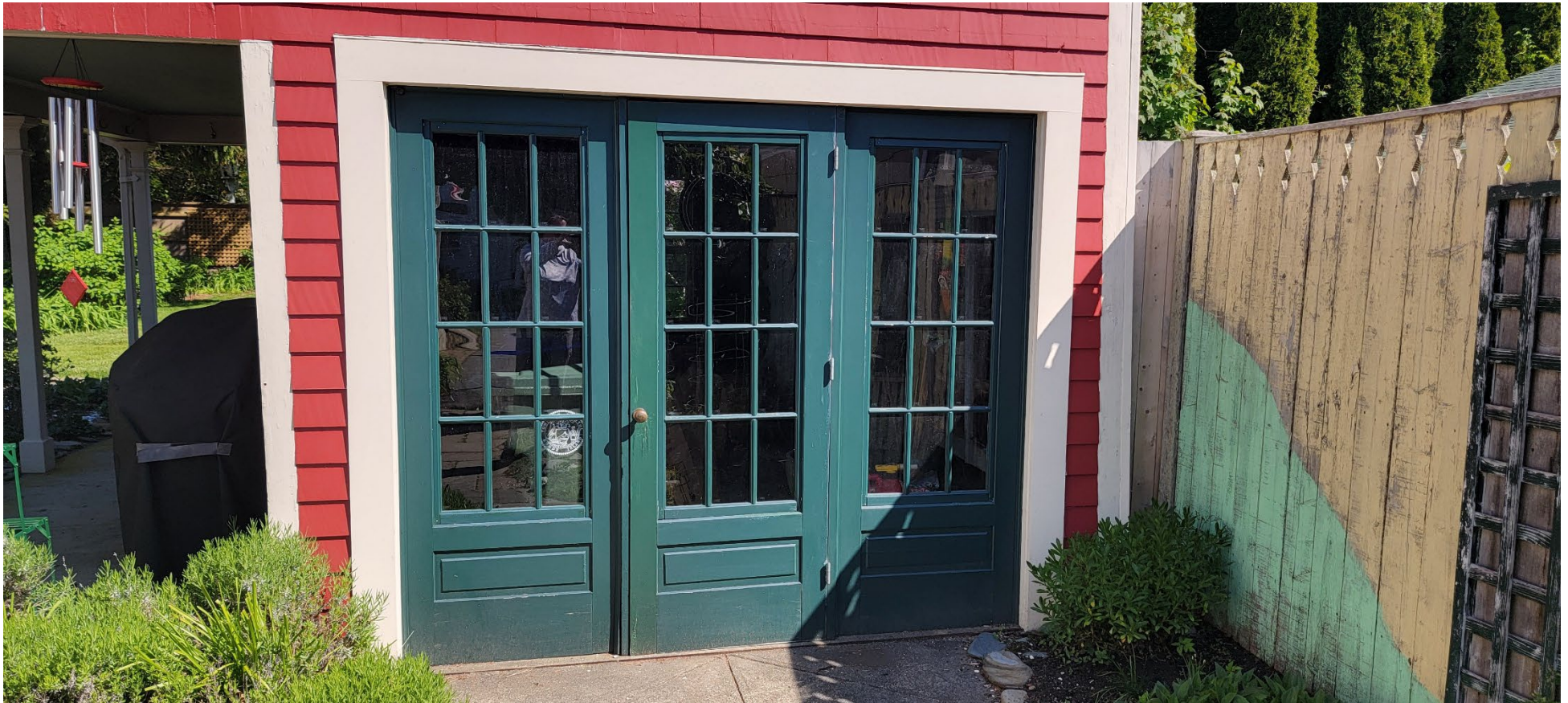
Photo #4: Main door at South Façade (triple set of 12-lite French doors)
