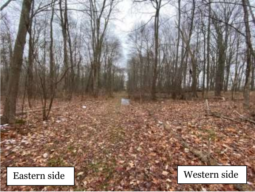
Photo 1: Depicting cleared sewer easement - 12/15/2022
