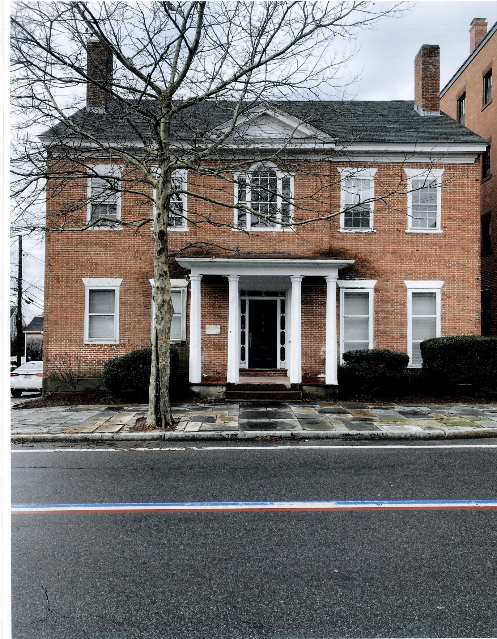
Hope Street façade unchanged other than new windows
