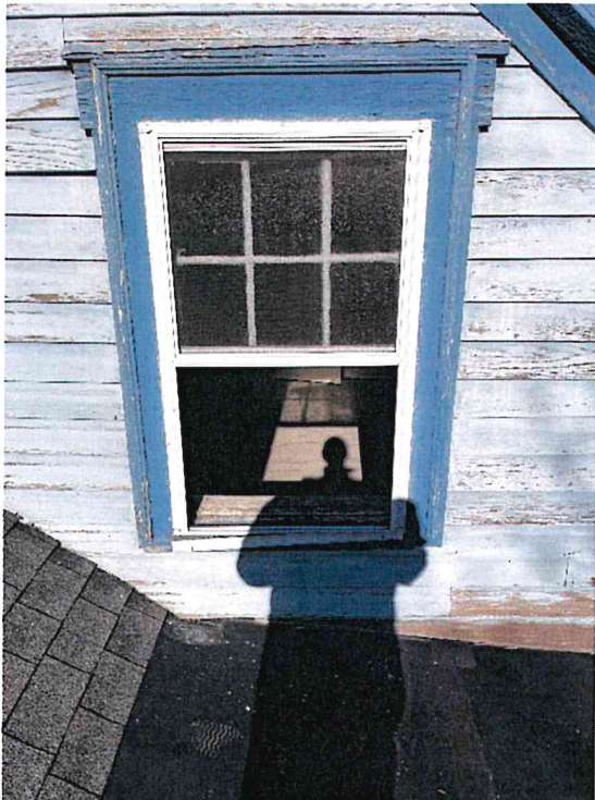
28 x 46 window 3 rd floor rear- Propose to change to casement- See spec on page 17
