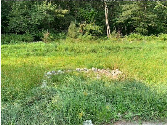
Photo No. 2: Vegetative growth within PWW
