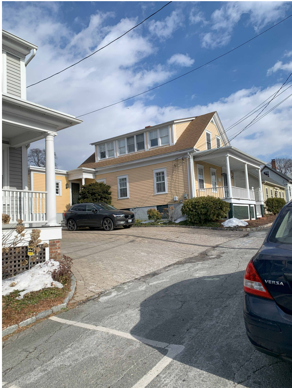
Photo #2: Front West side view, southwest corner of property
