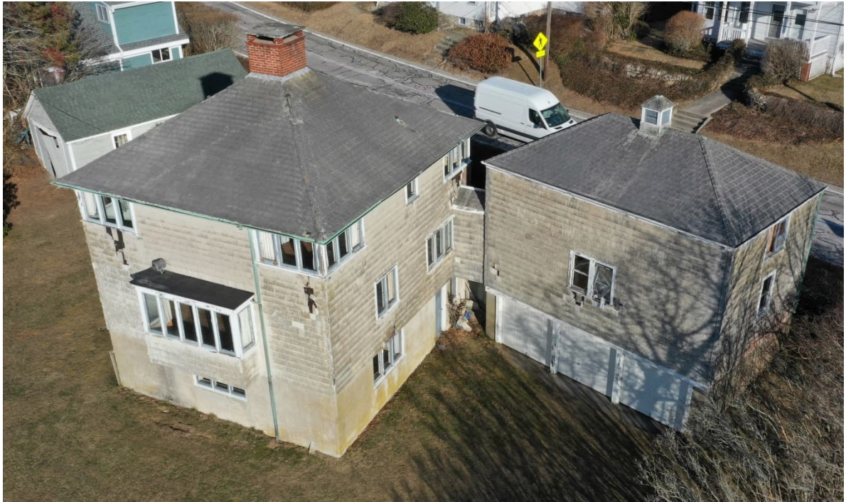
Overall aerial photo of 125 Hope Street taken by WSP with a drone looking approximately north.
