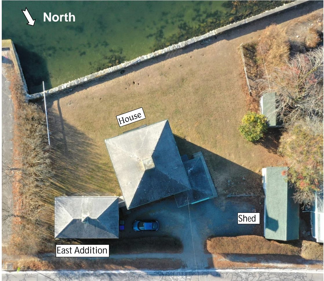
Overall aerial plan photo of 125 Hope Street taken by WSP with a drone. North is oriented approximately down on the page.
