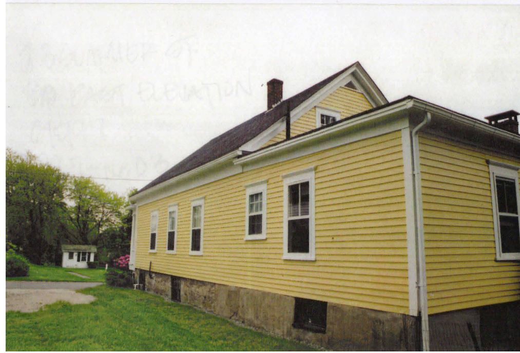
Photo #6: South & West elevations, 06/05/1997
