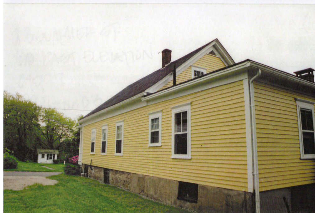
Photo #6: South & West elevations, 06/05/1997
