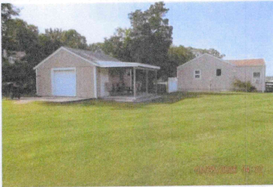
Cottage & Garage - to be demolished
