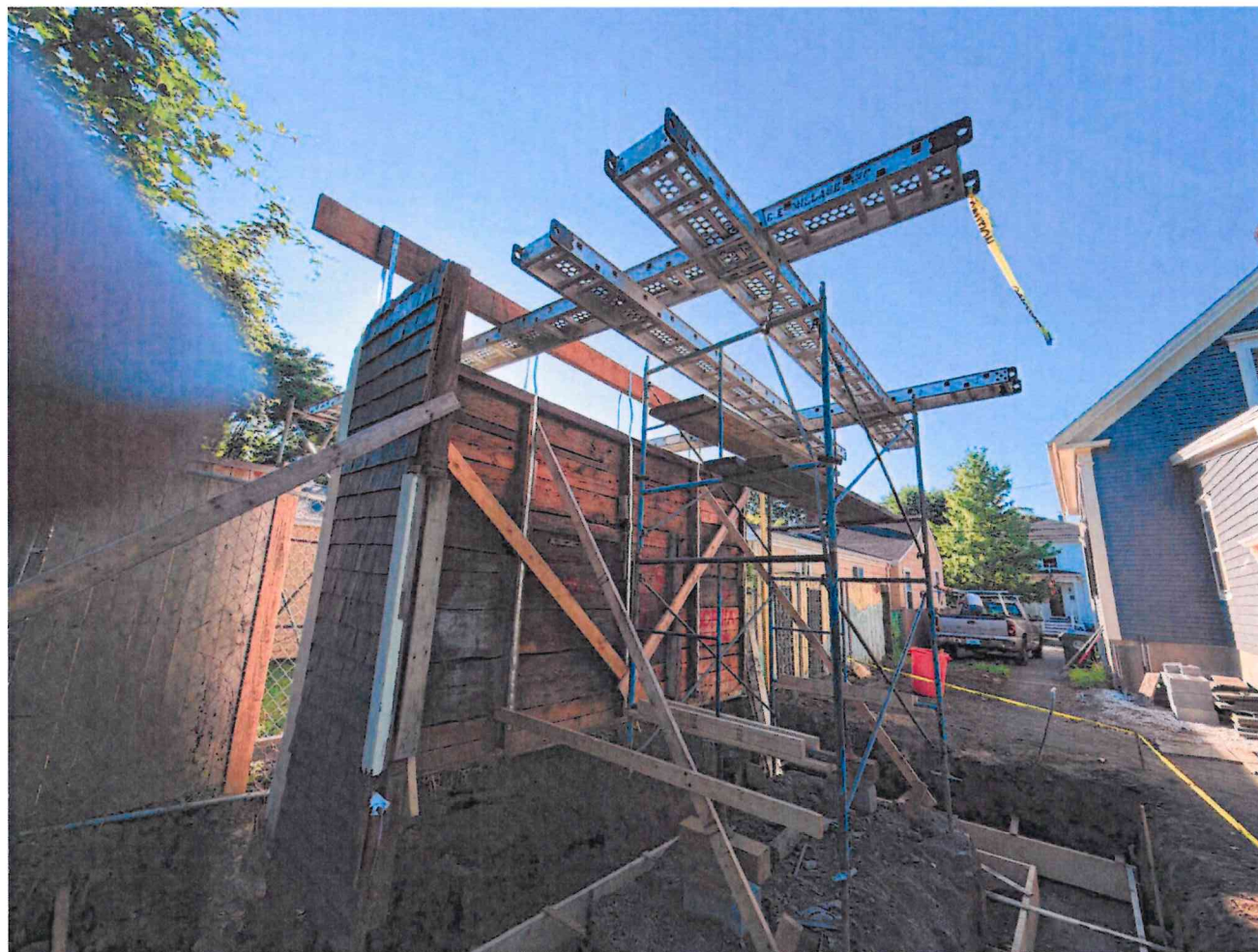
Scaffolding structure used to maintain existing walls in place
