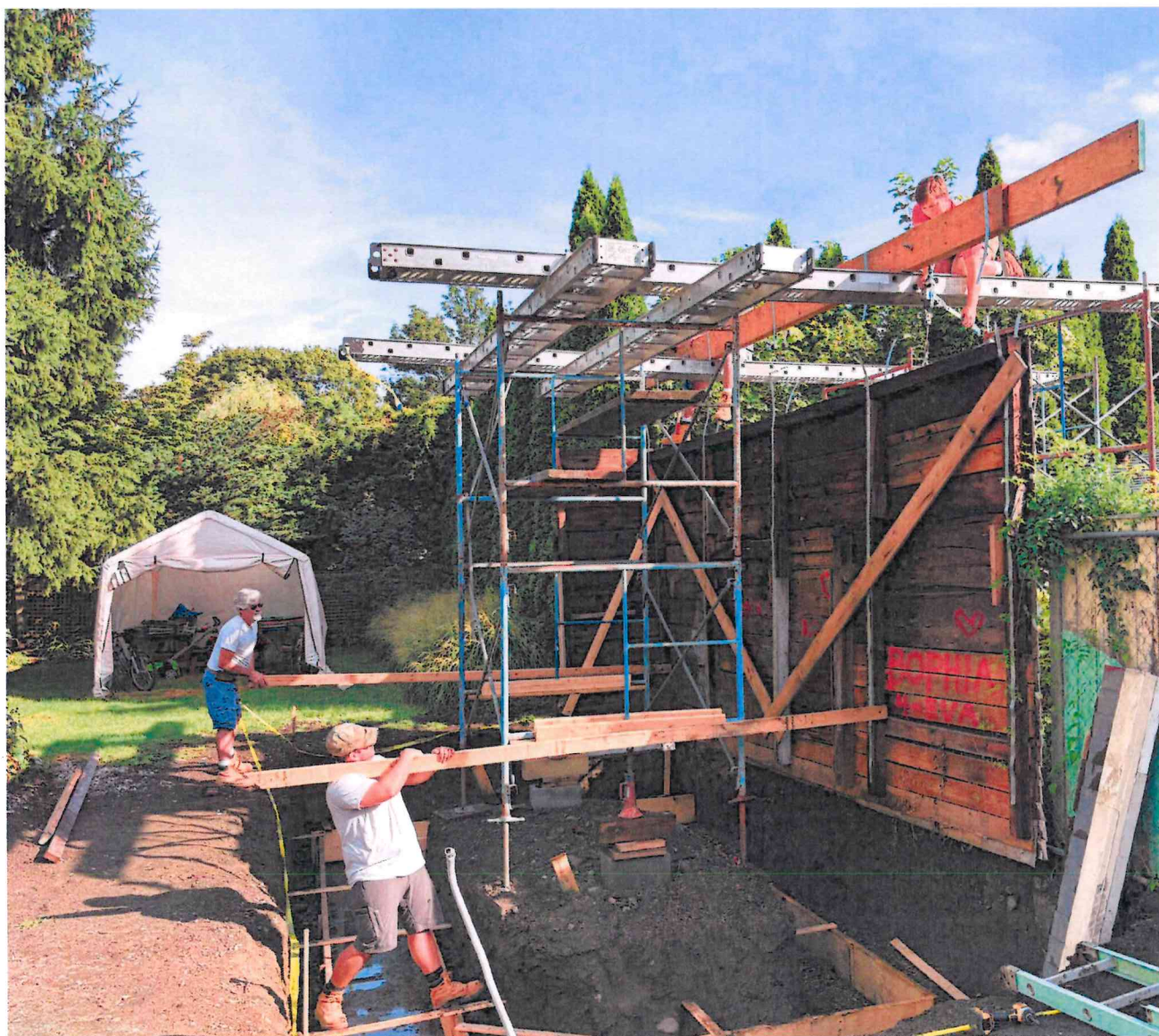
Scaffolding placed to support existing East wall (to the right)
