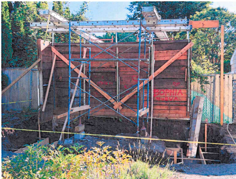
Existing East wall as viewed from the backyard
