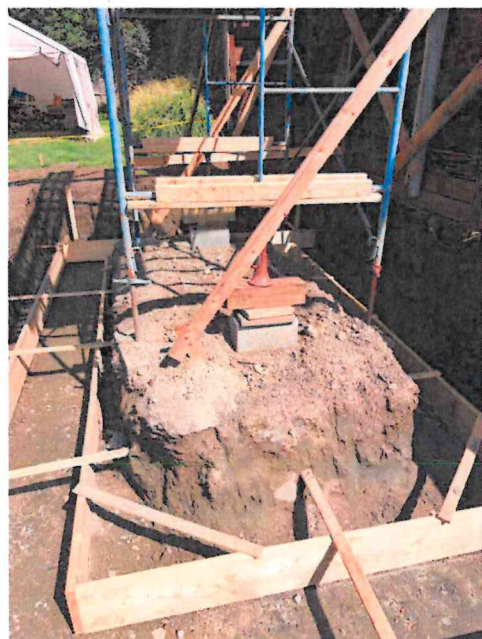
Excavation for footing
