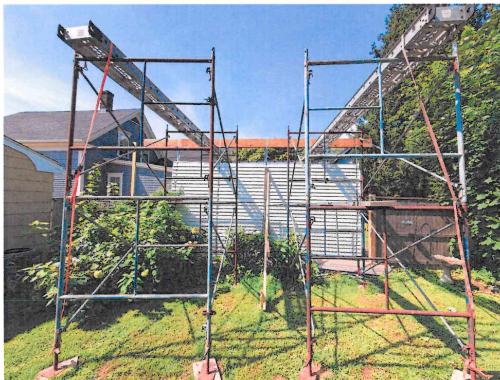
Existing East wall as viewed from the neighboring property
