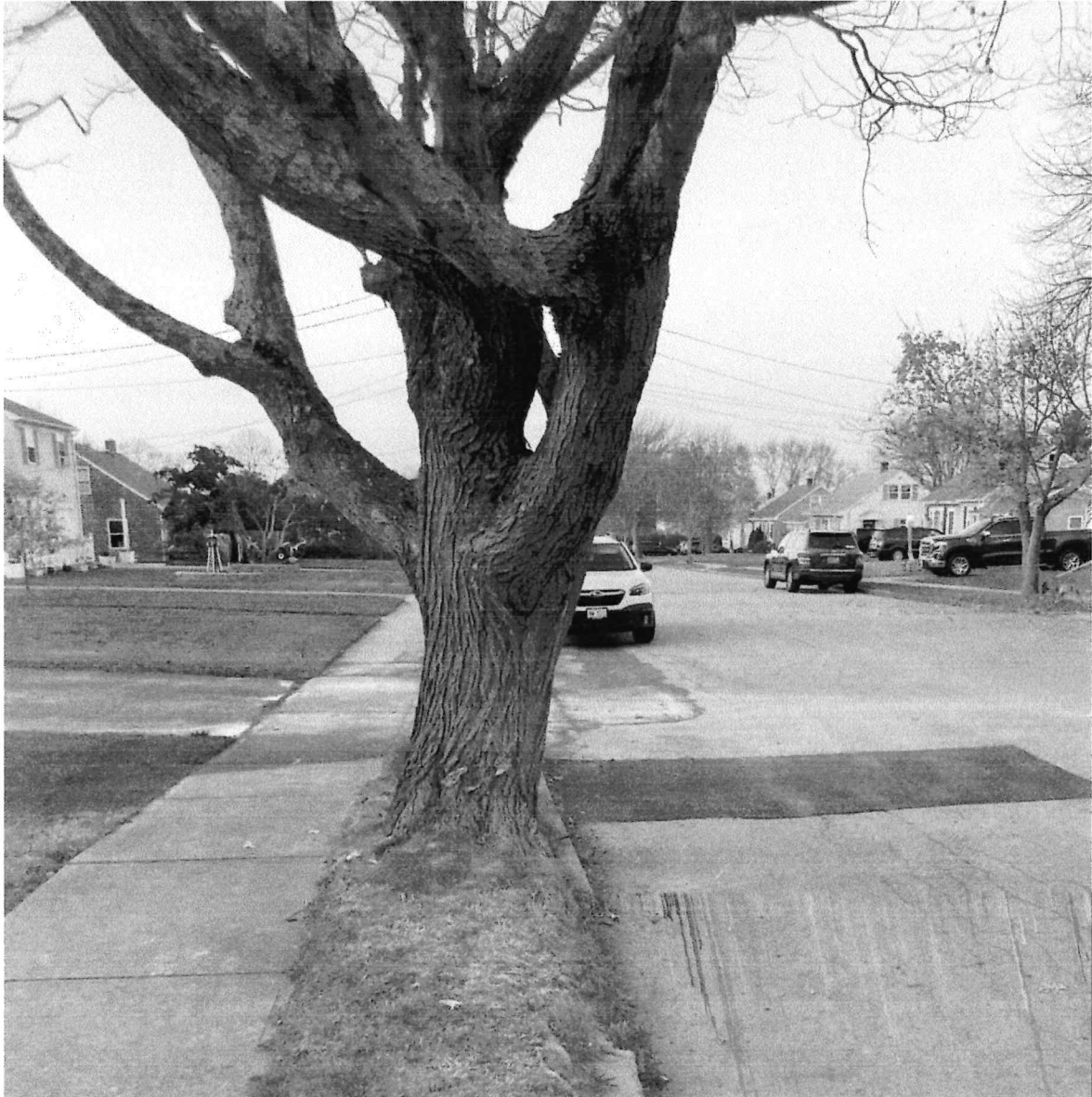
Tree and where the line was replaced
