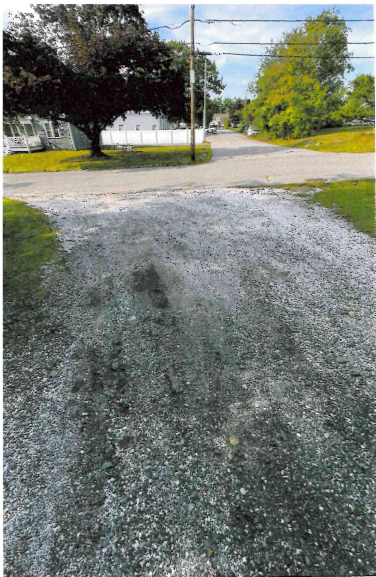
Hilltop - North toward Tower Road
