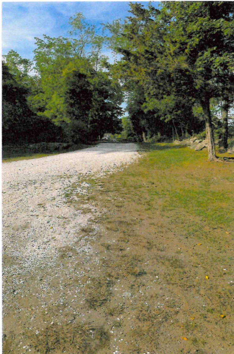
Hilltop Road @ Northeast corner of Lot 53
